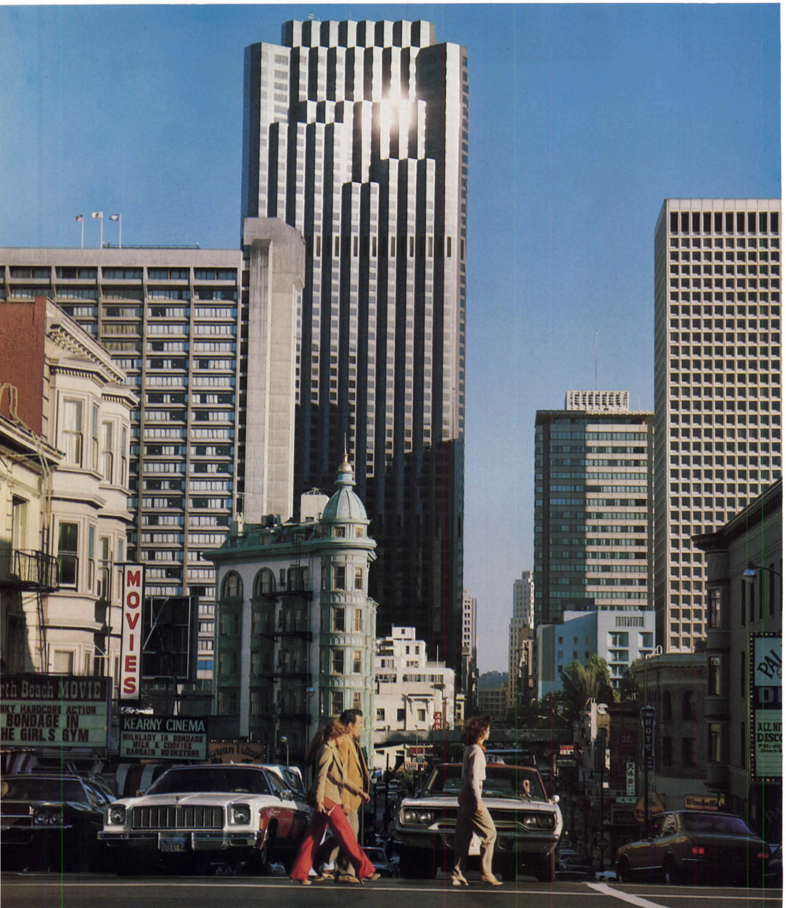
Even from skyline perspectives, the Bank of America's facade serrations are prominent in raking sunlight. The setbacks of its crown relieve the effect of the building's great bulk.
