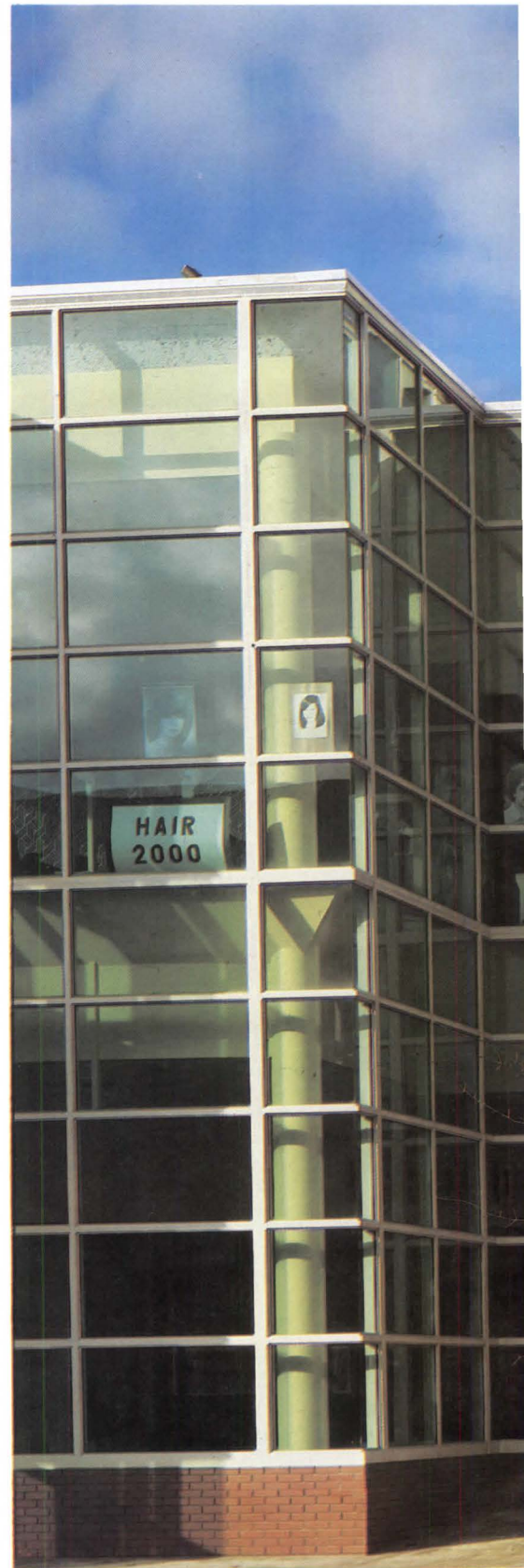
An elegant, second story glass and steel bridge links the mall and garage whose stair towers are glazed for security purposes (left). Though it lacks a curved stair, the Fourth Street entrance resembles that on Third. Both have bright red entryways that look like squared bull's-eyes.
