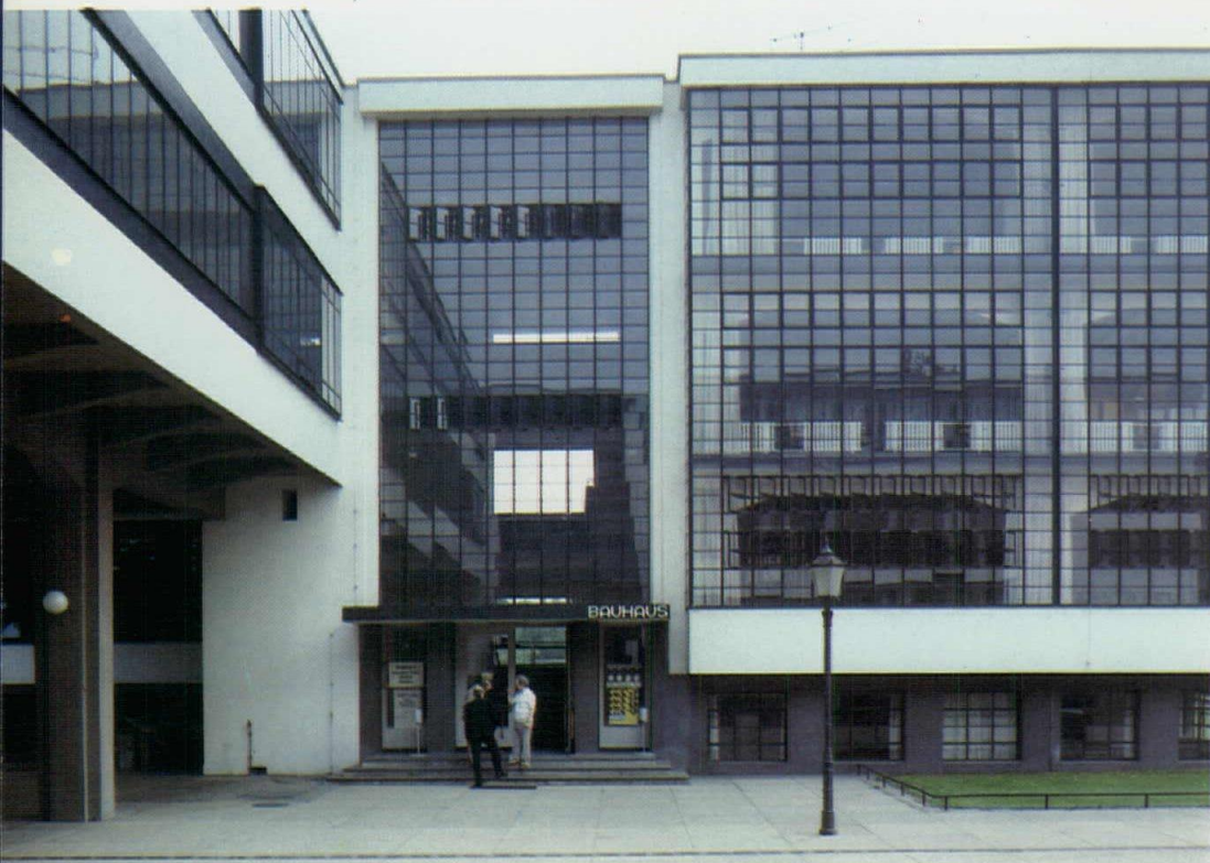
Left, entrance to the workshop wing and auditorium; the concrete structural system is visible behind the curtain wall. Top, bridge connecting the technical school on the left to the workshop wing; the architecture department was located on the top floor of the bridge with administrative offices below. Right, studio wing with 28 rooms, each with its own balcony.
