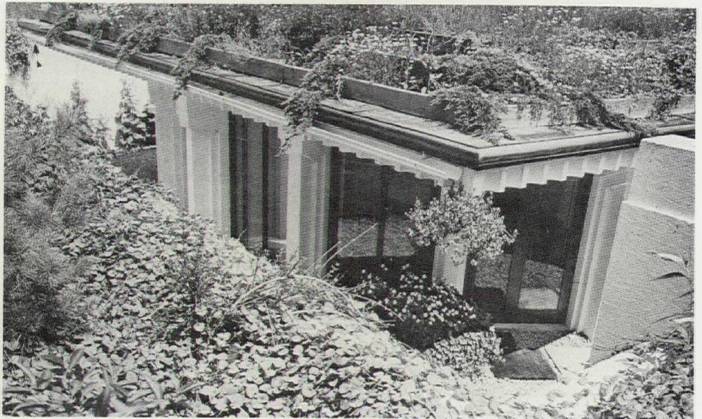
Wells' second office and his first underground building, Cherry Hill, N.J. (1970).
