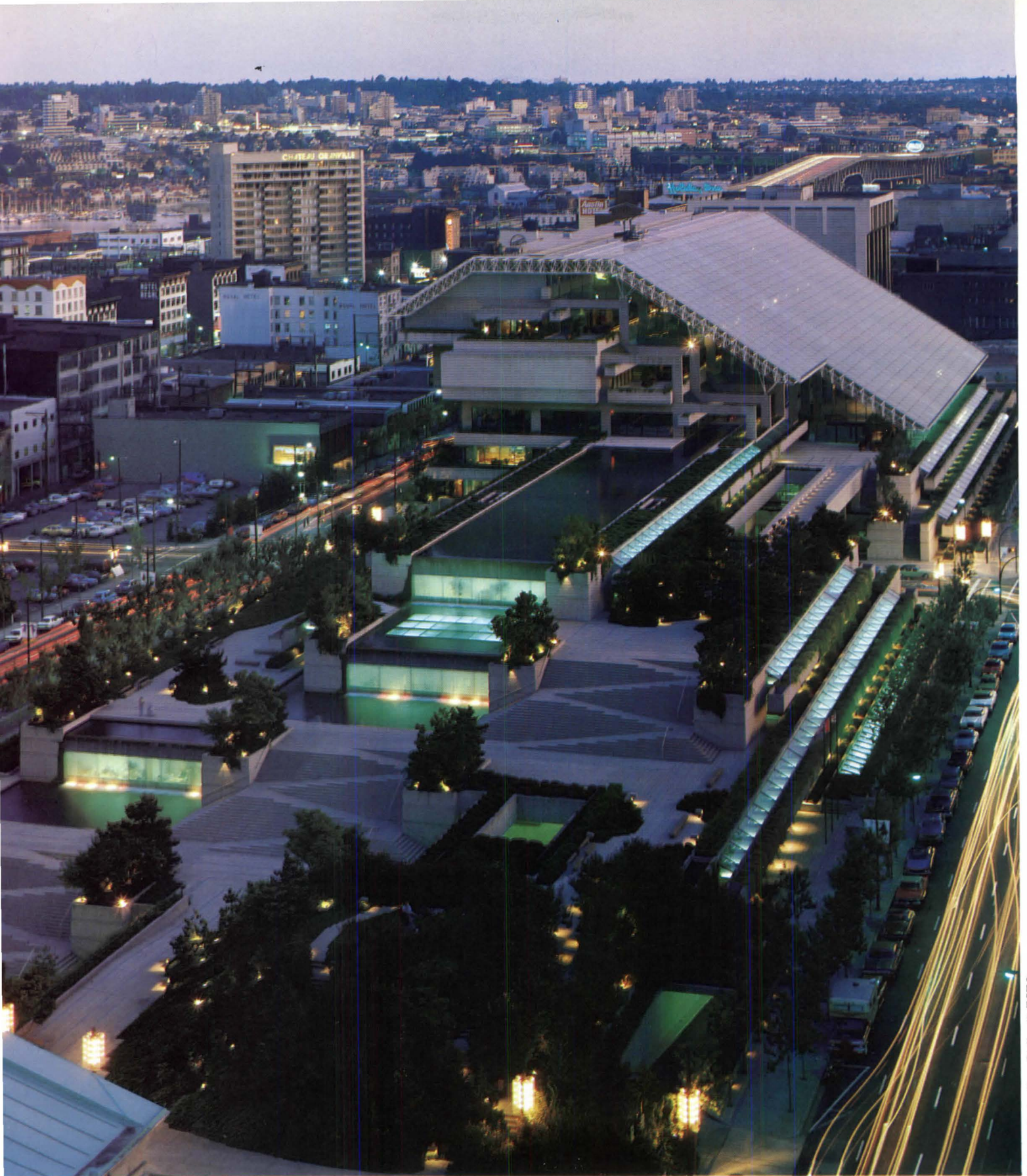
Photographs by Ezra Stoller © ESTO
