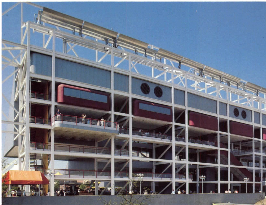
Above, the U.S. pavilion's sloping north wall of foam-filled steel panels and insulating glass. Left, its Beaubourg-like southern side, with exposed steel cage inset with escalators, stair towers, elevator shafts, balconies, and office pods. Facing page: above, solar powered telephones and a view through a cluster of international pavilions on the grounds' north end, and below, along the Waters of the World toward the Sunsphere at twilight.
