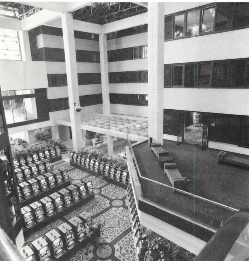
The Tropicana was built around the skeleton of the former Ambassador Hotel, which had not been occupied since 1968. Its atrium mezzanine (above) is now packed with slot machines.
