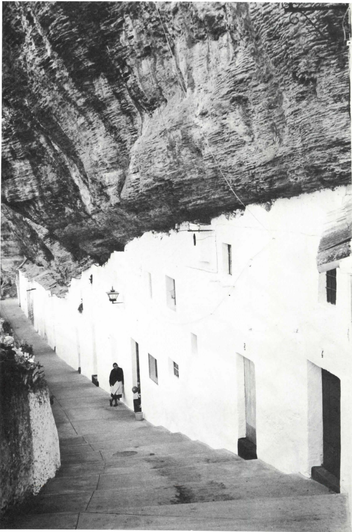
Across page, near the town of Baza, a cave house with white-washed openings and red peppers hung out to dry. Above, the village of Setenil grew from a collection of ancient cave dwellings along a river. Facades have been built in front of the caves offering a more conventional image of 'home.' □
