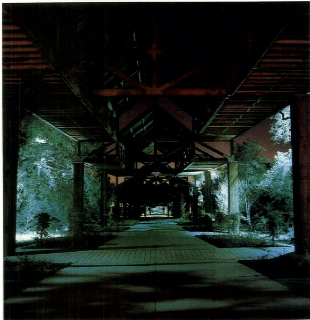
The pergola contains no lighting itself, but is lit from mercury vapor downlights hung in nearby trees.
