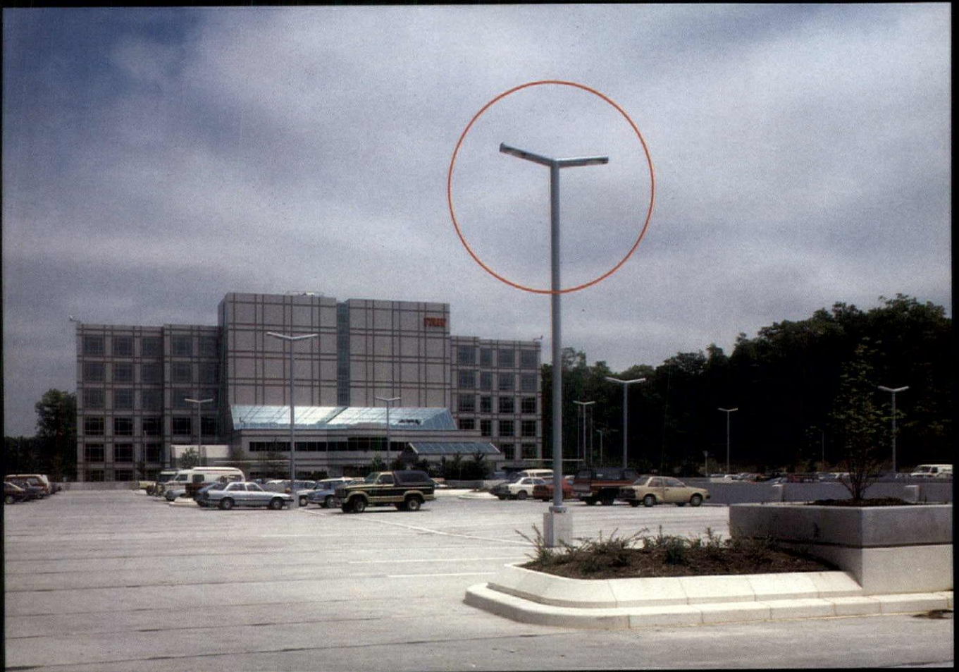
TRW Building, Fairfax County, Virginia
