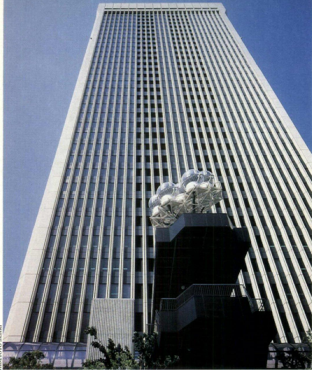
Perched atop the roof of an open-air staircase, this seven-unit cluster catches the day's sunlight and transmits it to the building's interior.
