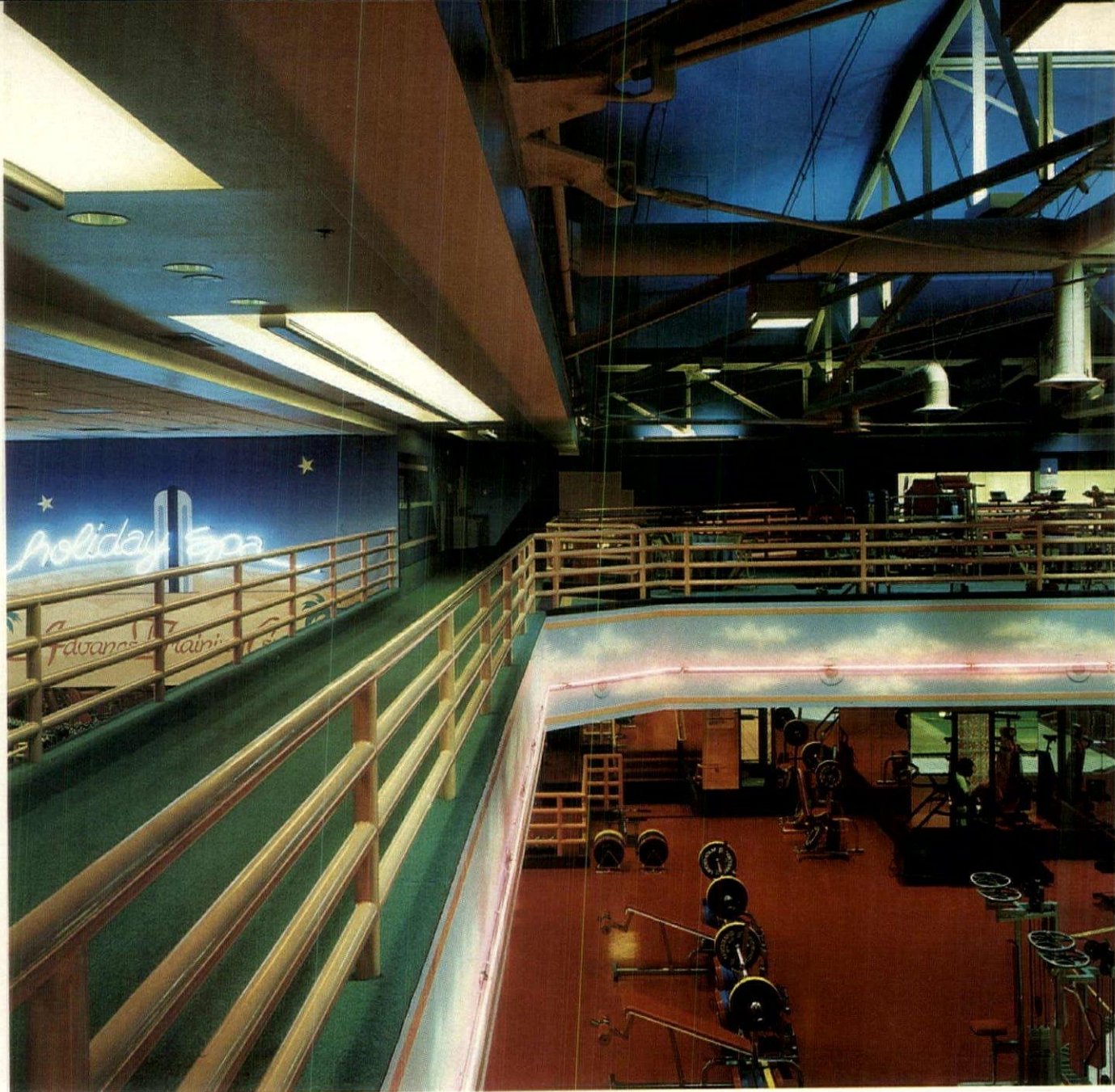
Indirect fluorescent lighting prevents glare from distracting runners on the one-eighth-mile track.
