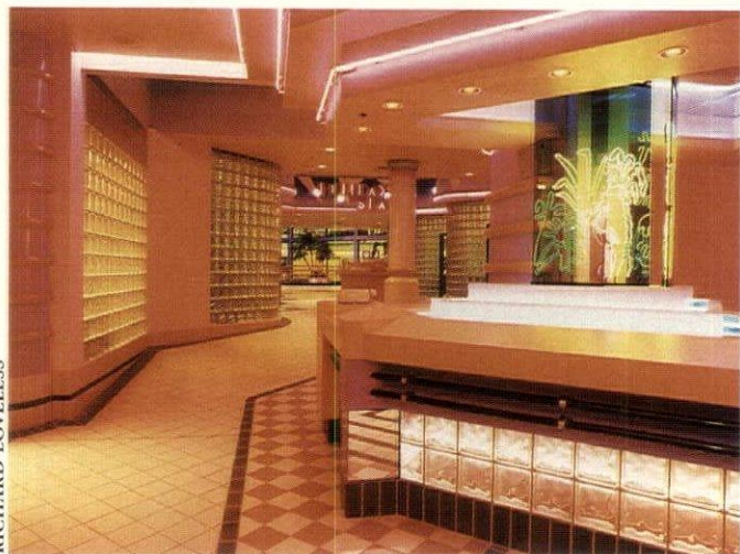
Recessed metal halide downlights light the entry stairs and forward lobby. Glass block walls of nearby offices also contribute light to the lobby.
