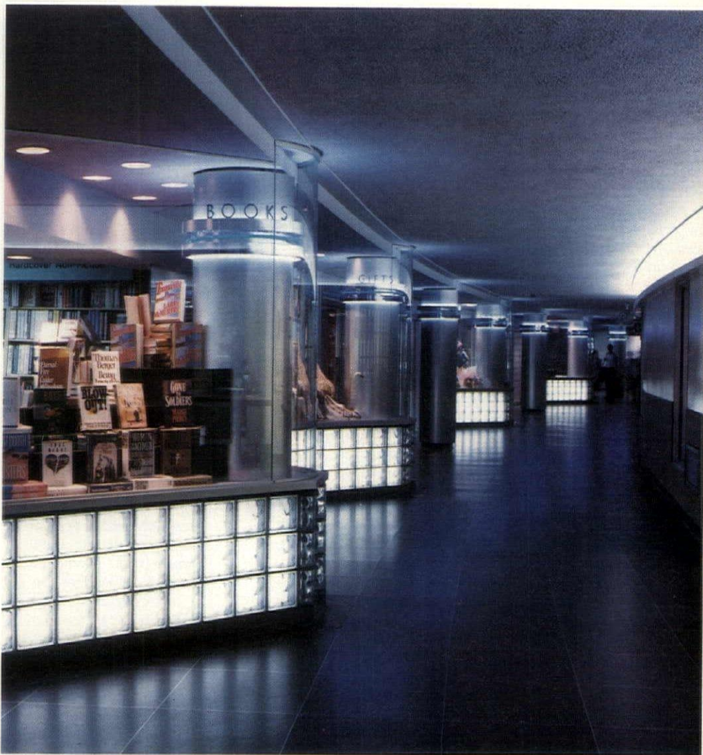
New glass block walls and cove are lit with concealed cold cathode.
