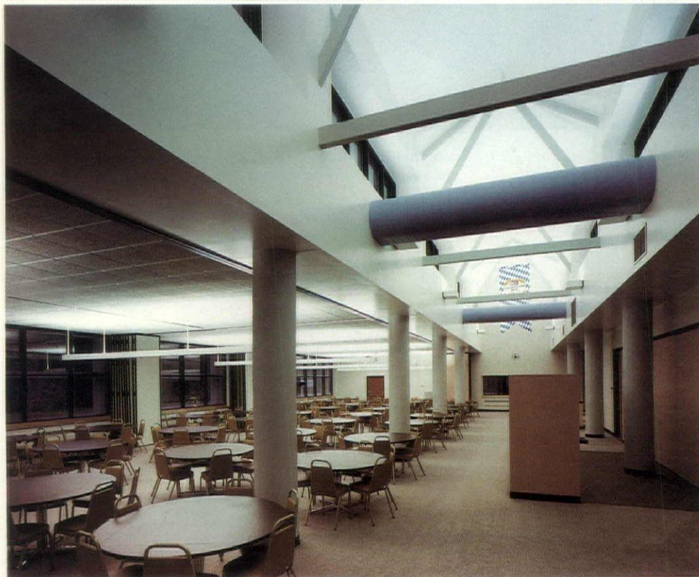
Ten 250-watt metal halide uplights illuminate the 24-foot-high clerestory to provide an average of 20 footcandles on surfaces in the 18- by 90-foot central service area directly below. The uplights draw attention up to structural elements and banners in the clerestory and provide general nighttime lighting levels similar to daylighting.
