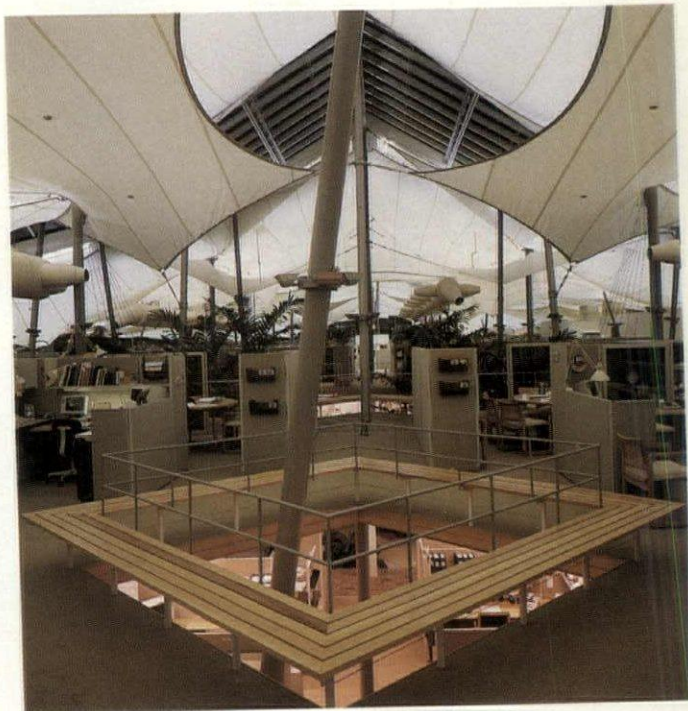
The sophisticated tensile structure at the Bradford Exchange, left and above, disguises an unsophisticated lighting system — fluorescent strips applied to the roof of a metal building.
