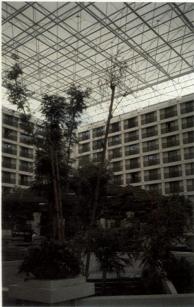
A fiber glass fabric structure atop the atrium at the Hyatt Regency Hotel in Burlingame, California, provides soft, spectrally balanced daylight for plants and people below.
