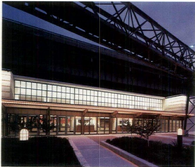
UNION STATION 10 CINEMA is nestled under Highway 40 in St. Louis (above). Recessed incandescents graze piers (bottom). Double-thick concrete walls and 8 inches of concrete on the roof block highway noise inside.
