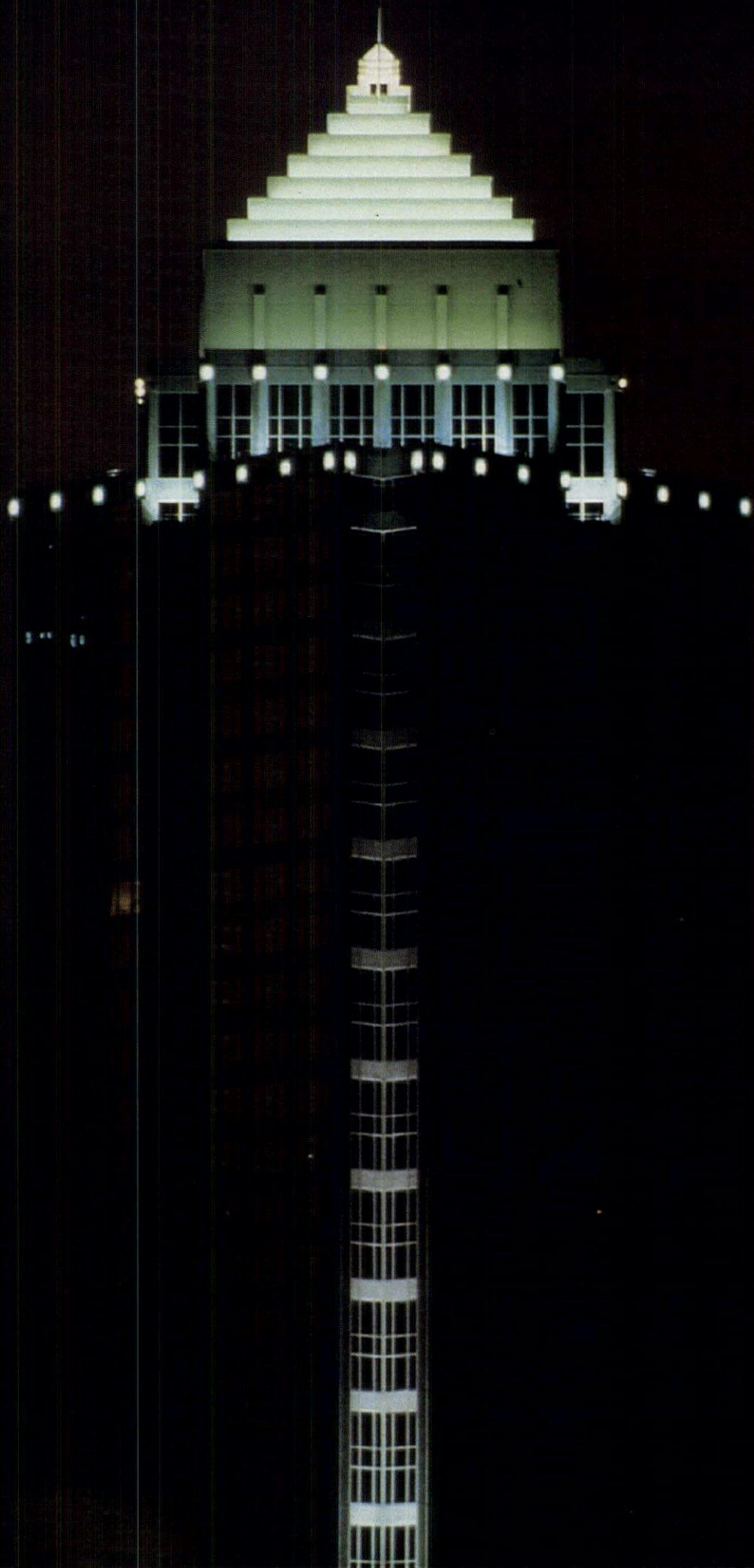
SKYLINE BEAUTY: The pyramidal roof structure is connected visually to the rest of the building by shafts of light shooting up the reentrant corners.
