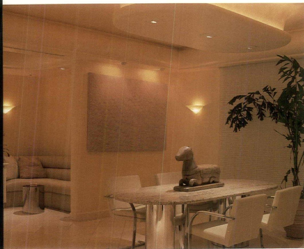
HUMLESS DINING: (Above) The thicker glass envelopes of the A19 rough service lamps in the sconces reduce filament hum when the fixtures are dimmed.
