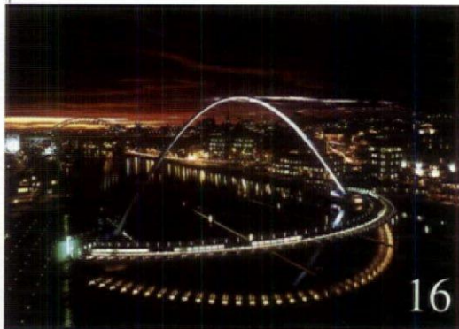
GATESHEAD MILLENNIUM BRIDGE
