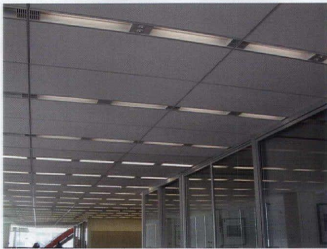
The dual-lamp ceiling fixtures (above) have a multi-purpose center area to incorporate sensors and sprinklers, and the end compartments take the air return back into the ceiling plenum. The result is a clean and tauged ceiling plane of light slots. Shades on the different elevations of the building respond to the daylight conditions at the southwest corner of the mock-up, while sensors mounted to the ceiling and the floor take illuminance readings (left).
