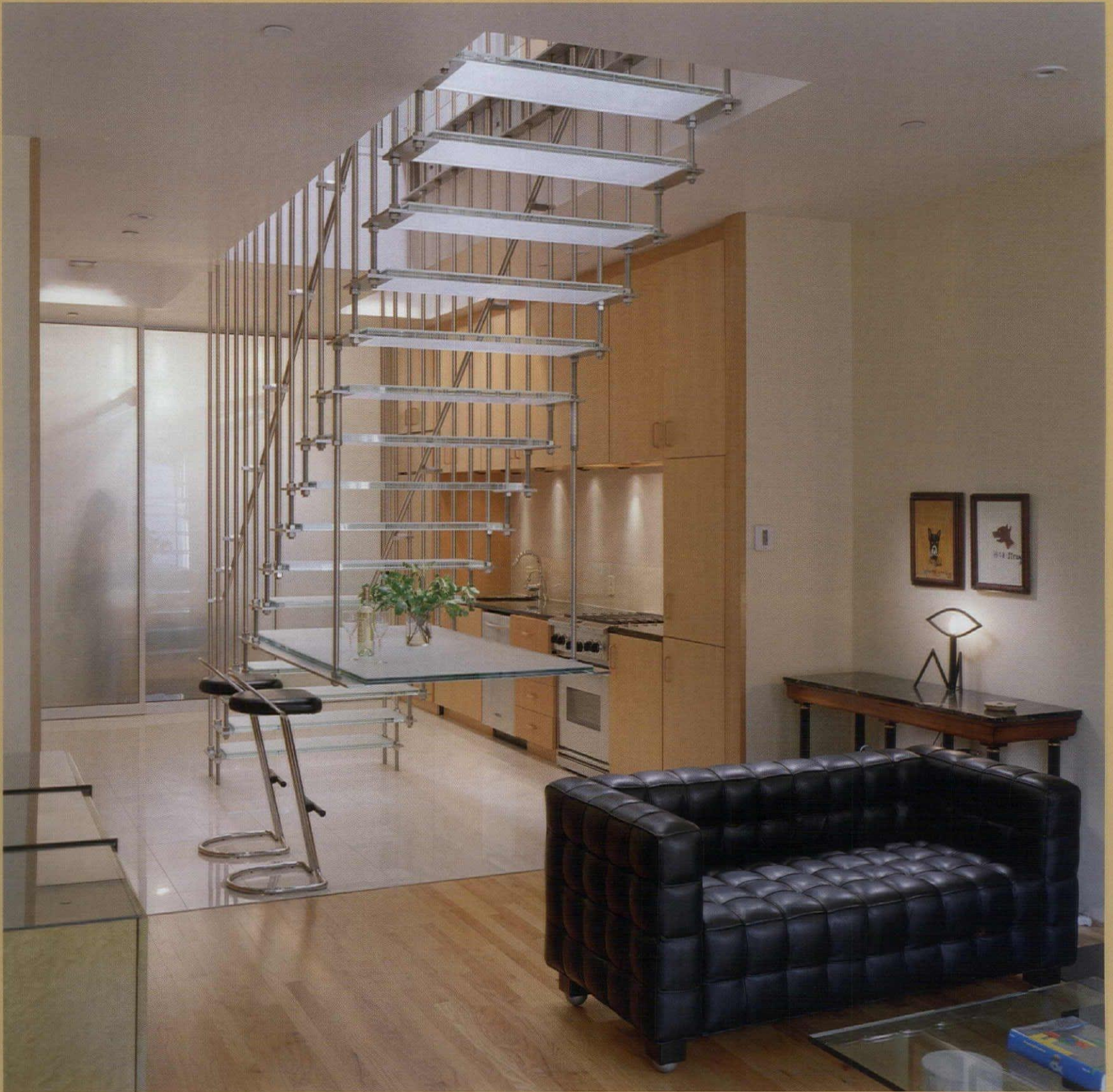
Plan diagrams (below) and an east-west longitudinal section (facing page) highlight the loft's glazed openings and the path and intensity of daylight that enters the apartment. The loft's focal point—an open-tread glass stair—allows light from a skylight above to fill the lower level and provides a unique backdrop for the kitchen eating area (above).
