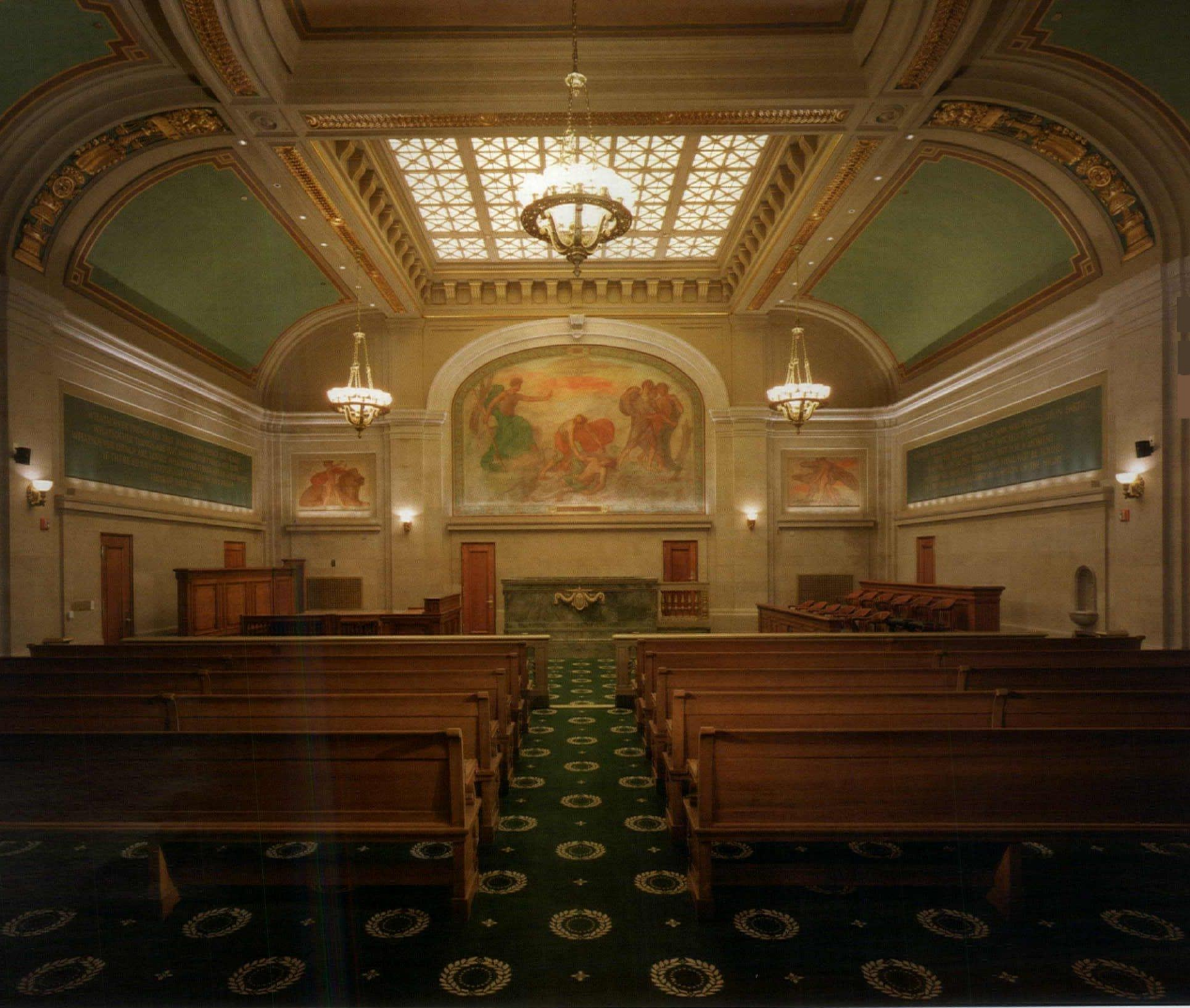
A variety of spaces enabled different types of illumination to supplement existing systems. The most diverse is the Codey Courtroom, which includes an internal laylight backlit with fluorescents, historic filament lamps in the restored fixtures, and MR16s to highlight word panels on both sides of the room (above). (Only half of the lamps were illuminated in the above photograph.)
