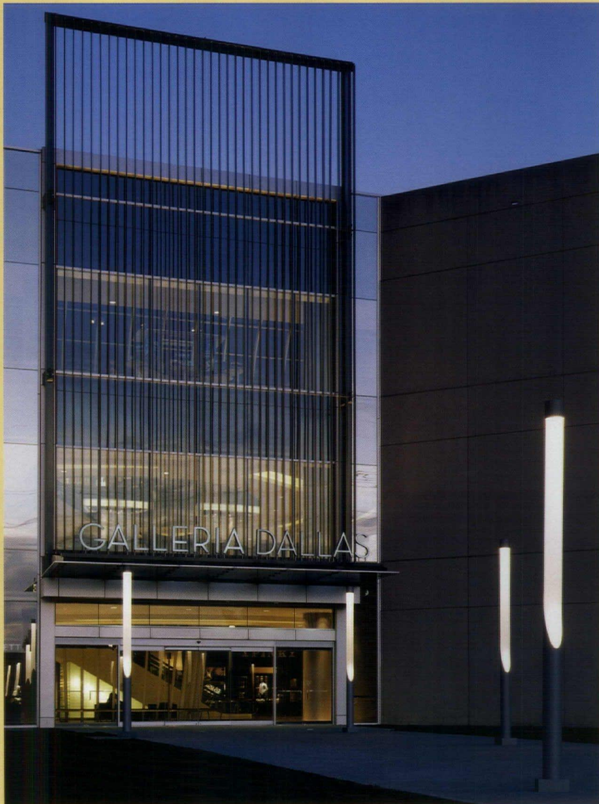
The entrance to the recently renovated Dallas Galleria is defined by a window-like curtain wall, covered with a breeze soleil and a procession of column luminaires (above). Inside, the vaulted skylight creates a backdrop of daylight, providing the first layer of illumination (facing page).
