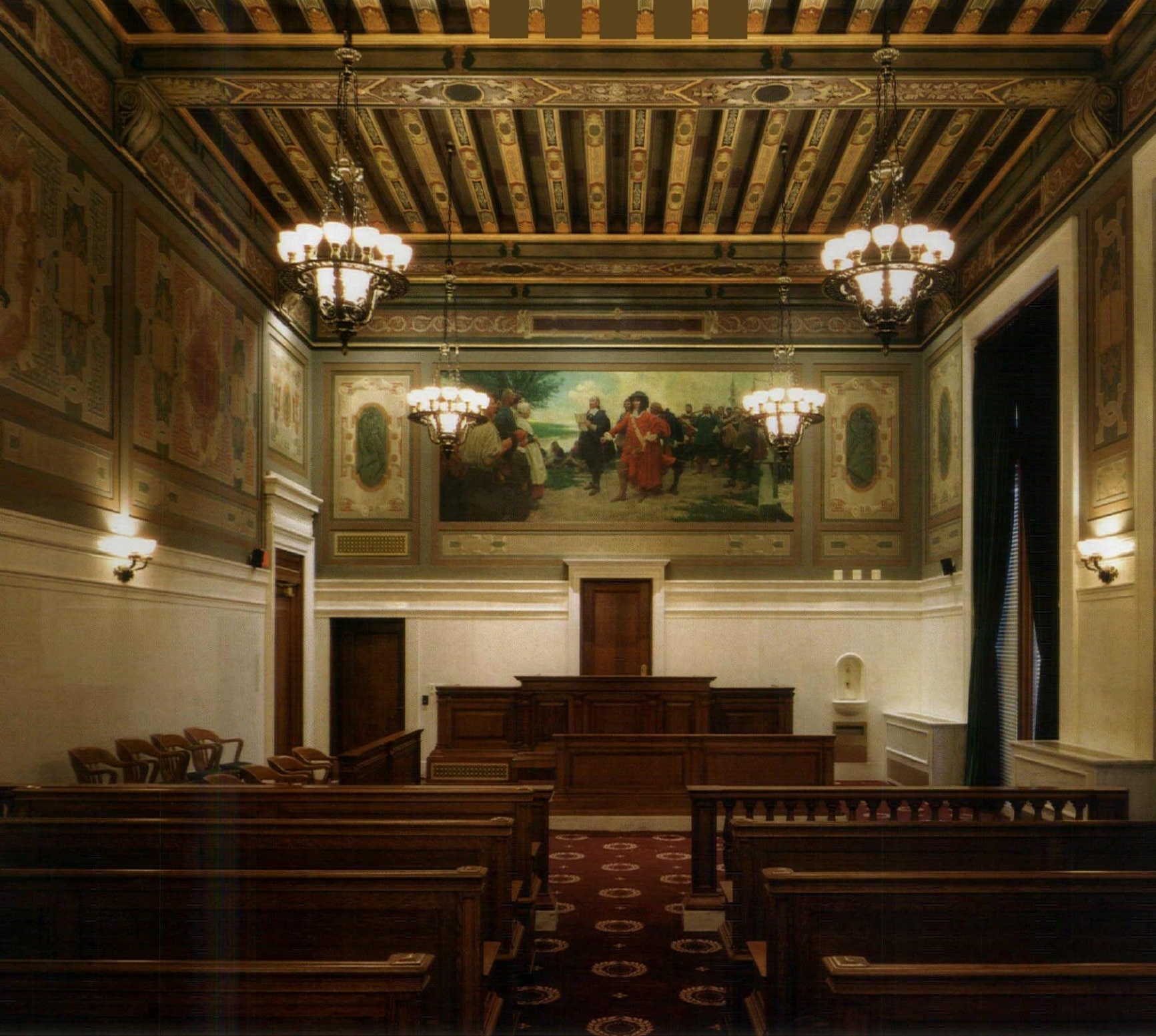
In a courtroom with an elaborate Venetian-style ceiling, the main illumination is provided by chandeliers and wall sconces. Original pendants were modified to include a central glass bowl that houses additional lamps on dimmers (above). Lighting each level of the atrium's dramatic volume not only highlights the artwork, but creates an evenly illuminated space (following page).
