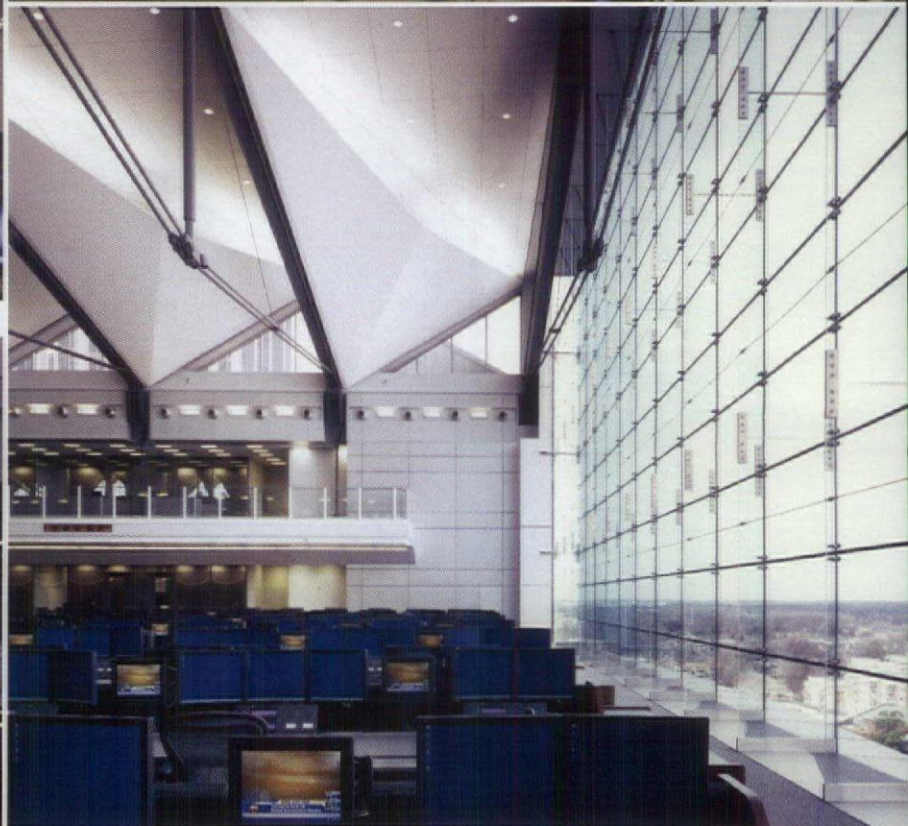
A 100-foot-long bronze-tinted Pilkington curtain wall anchors the north trading area. The perimeter of the space is flanked with continuous cove uplights, and the main ceiling houses ceramic metal halide recessed downlights (top left). A king-post truss system enabled the 50-foot-tall space to be column free, and to have clerestory slots that permit even more daylight to fill the space (bottom left). The folded planes of the ceiling are illuminated with T5 cove lights concealed at the top rim of the folds (bottom right). The 35-foot-high south trading area accommodates different trading requirements, and as such, is illuminated with recessed slot lights. Also in this area, operable aircraft hanger doors are accented with an abstracted shape and the illuminated appearance is the result of daylight (top right). The east-west longitudinal section describes the facility's mechanical and air flow/return systems (below).
