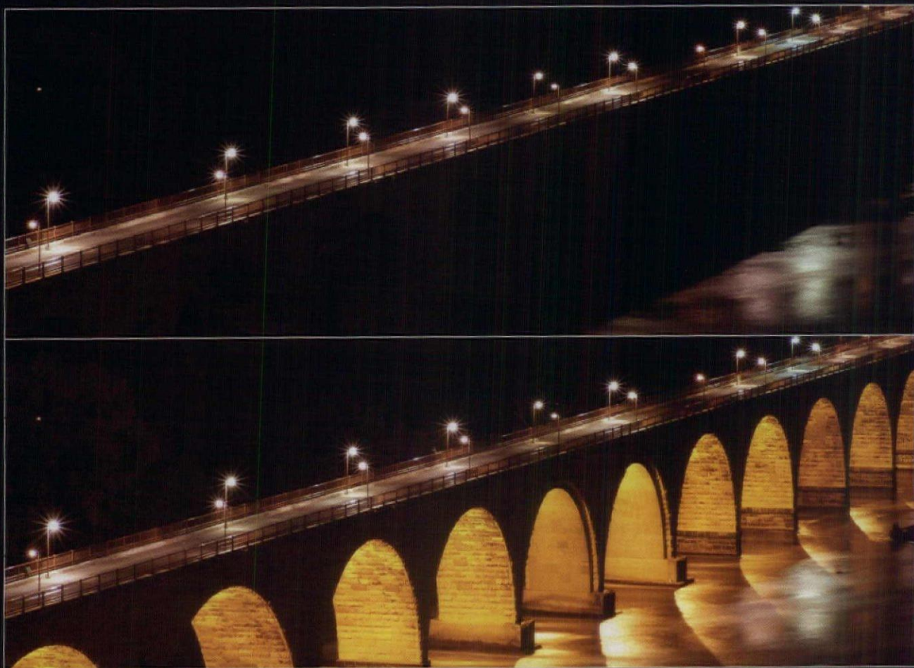
The Stone Arch Bridge now has a nighttime presence on the Mississippi River, and the difference between the bridge arches illuminated and not illuminated is striking. The color temperature of the light distinguishes between the upper pedestrian walkway, a cool white-blue light, and the undersides of the arches, which are washed with the warm tone of 400W high-pressure sodium lamps.
