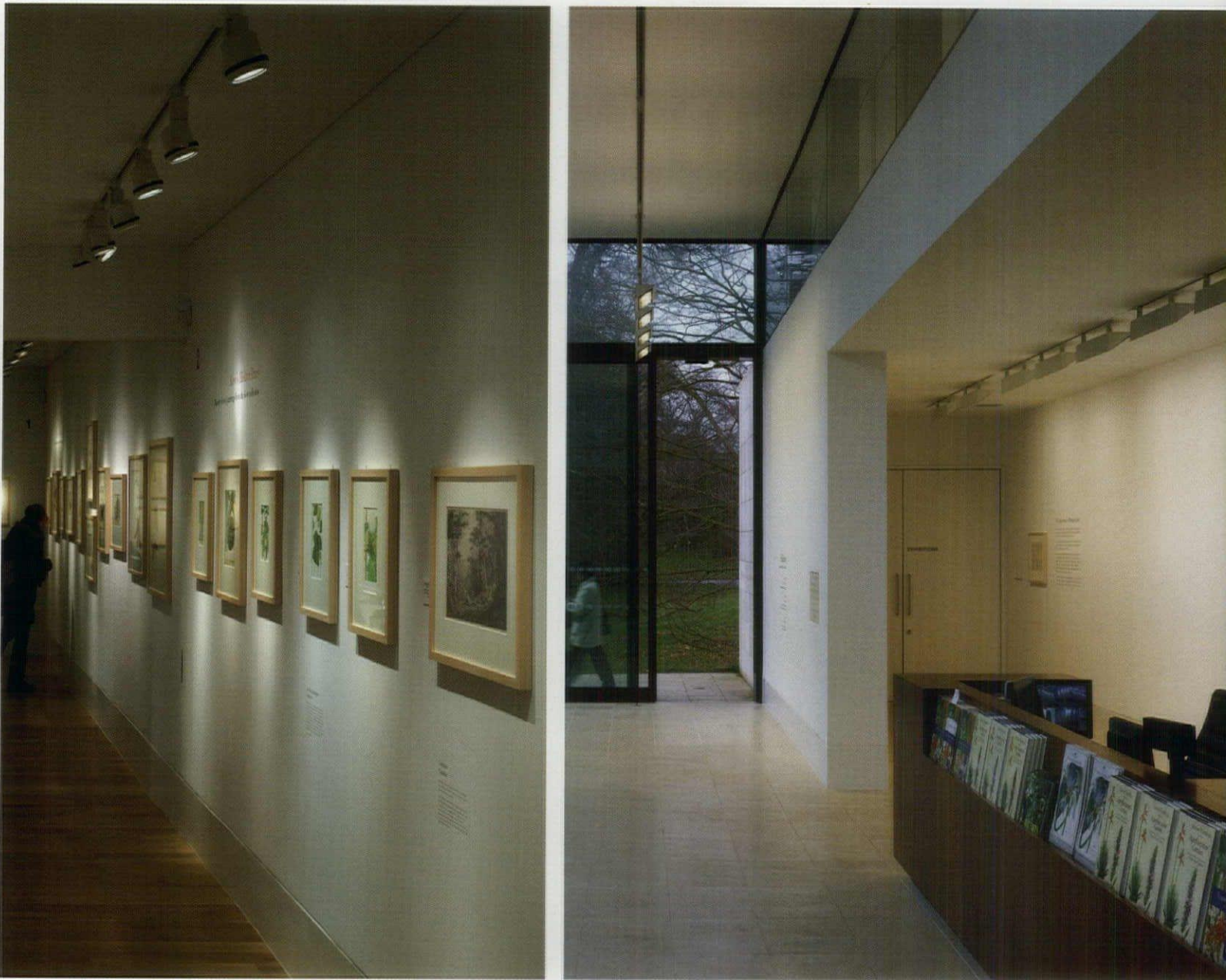
Tungsten halogen spotlights illuminate the Kew galleries (above left). The reception area is outfitted with track-mounted compact fluorescent wallwashers (above right).
