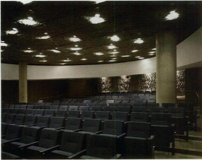
Architecture and lighting collide in the auditorium (left). Instead of grazing the hand-scrunched screen that lines the walls and ceiling, the lighting equipment is recessed behind the screen creating an uneven and patchy result. However, in the labs (right) and classrooms, lighting and architecture find a happier marriage in an integrated radiant ceiling system, based on a module of 10 feet, 5 inches.
