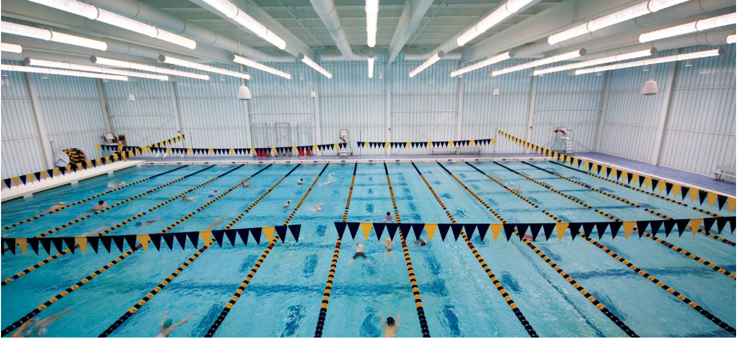
The main feature of the athletic center is the natatorium (above), which houses a competition-regulation swimming pool. The pool is lit with a light-pipe system that uses 1,000W metal halide lamps to provide the required 50-footcandle-level of glare-free illumination on the water surface. Metal halide downlights illuminate the surrounding deck areas.
