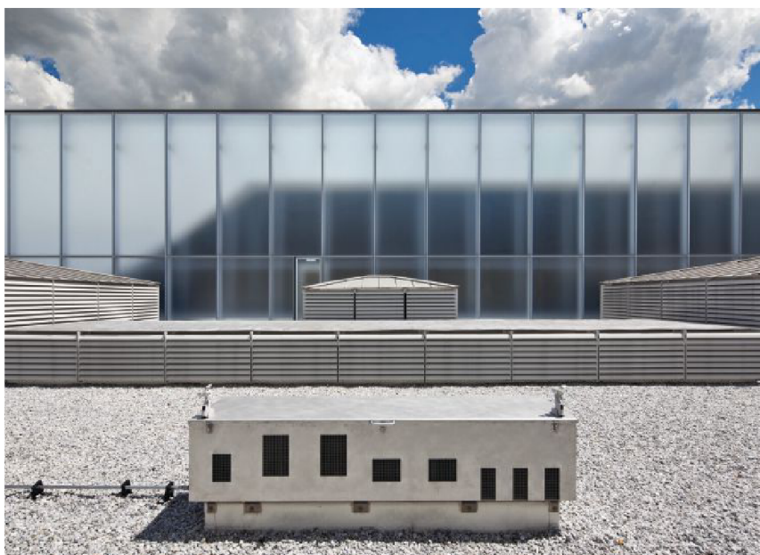
The Barnes Foundation at dusk (previous spread). A series of gardens and hard- and soft-scaped areas surround the museum. Visitors cross a reflecting pool as they enter the museum (top). A sensor on the roof—built as a miniature scale-model of the building—reads the galleries' light levels so that shades can be raised and lowered as needed (above).
