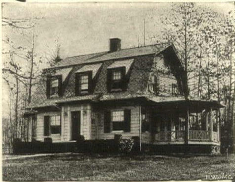
Residence of Mr. W. Hilt, Ridgewood, N. J. Covered with J-M Asbestos Shingles Ridgewood Development & Construction Co., Builders
