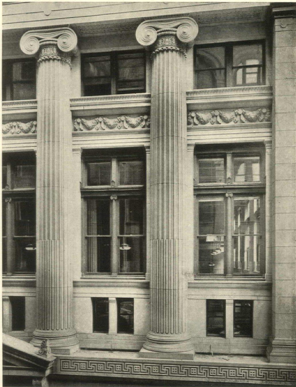
DETAIL, BANKERS TRUST BLDG., NEW YORK.
