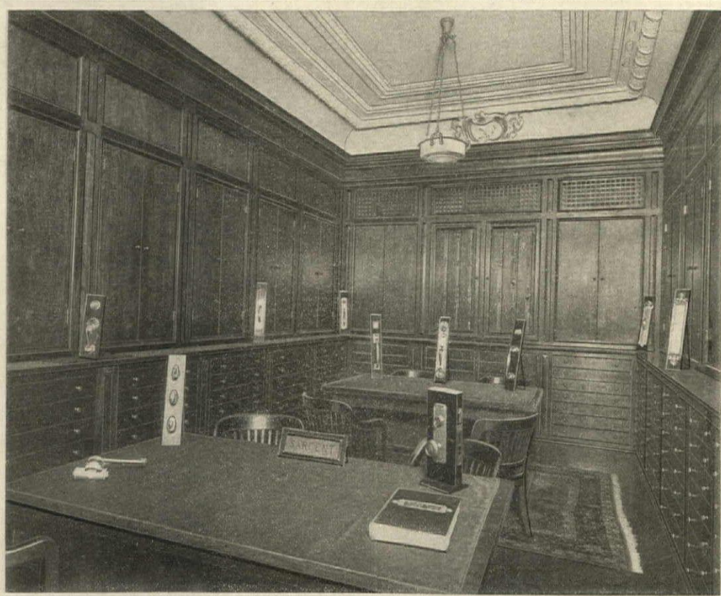
DISPLAY ROOM OF SARGENT & COMPANY CHICAGO
