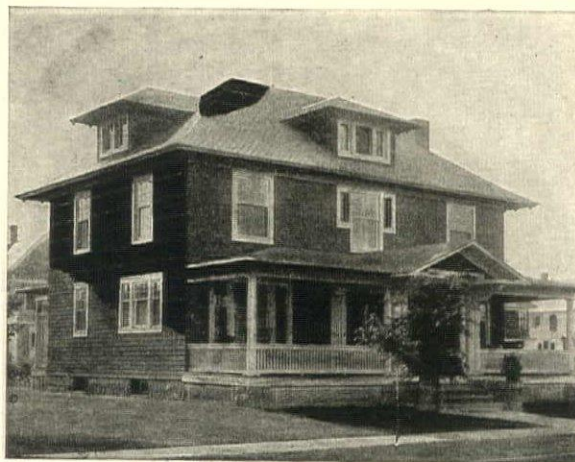
Showing Hydrex-Saniflor under clapboards.
