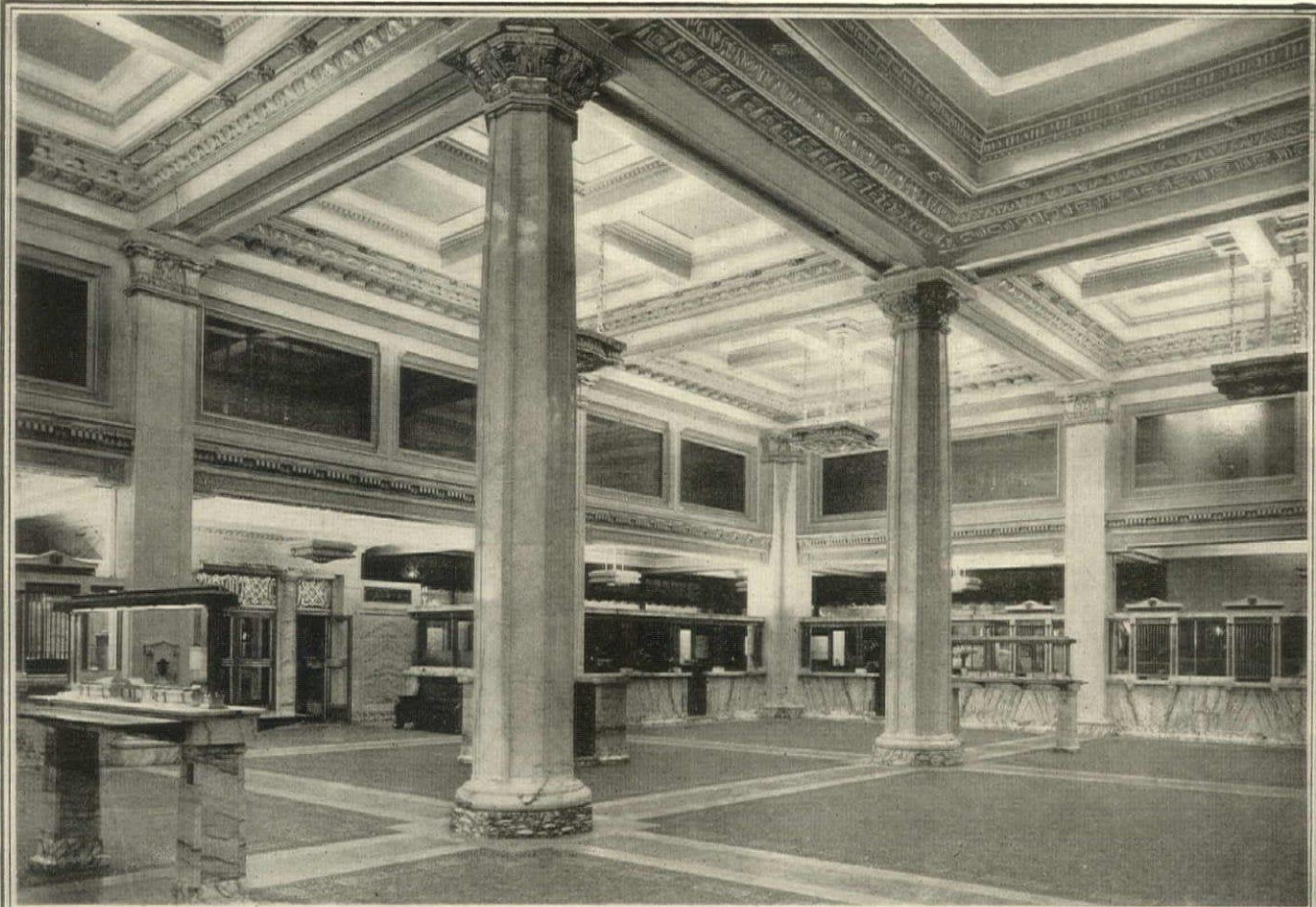
INTERIOR OF BANKING ROOM
