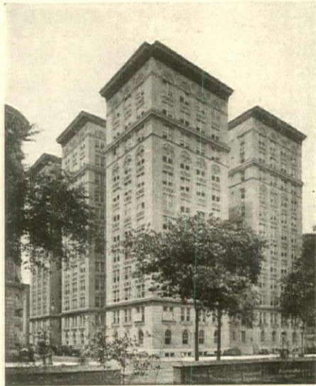
TURIN APARTMENTS, 93RD ST. AND C. P. W., New York. A. J. Bodker, Architect.
