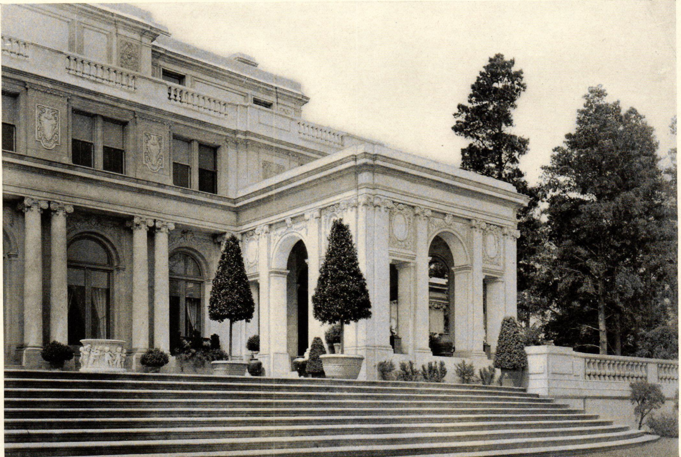
DINING LOGGIA AND ENTRANCE TO COURT.
