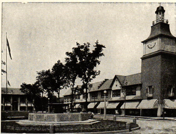
North Side, showing Sun Dial Tower and Fountain
