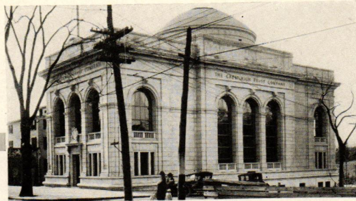
The Federal Granite Terra Cotta used for the dome matches exactly the granite used below.
