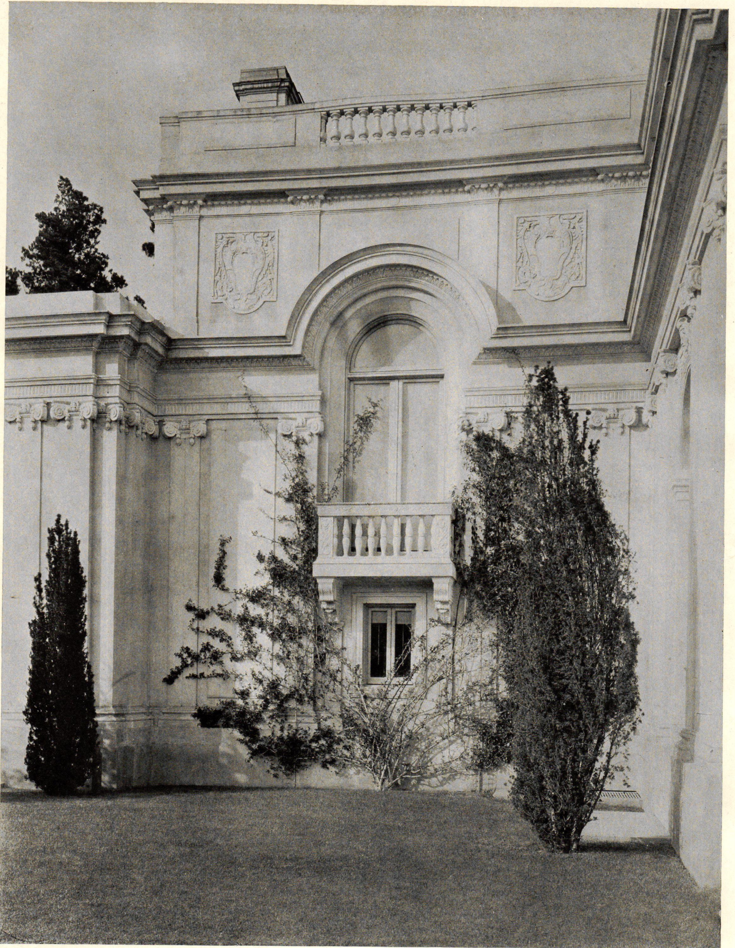
DETAIL, MAIN FAÇADE.
