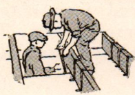
Hanging ceiling slabs
