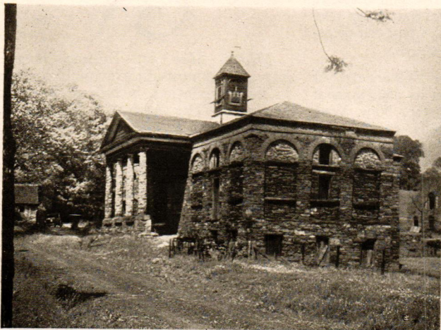
The stable of Bremo, built entirely of stone. It seems likely that it was intended to stucco the arched panels and the portico columns
