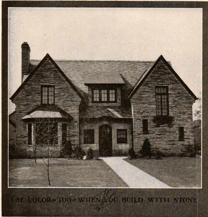
Howard C. Reep, Architect
