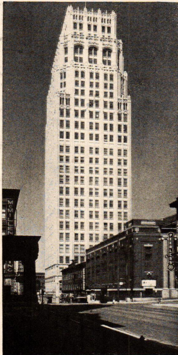
The Telephone Building, Kansas City, doubled in height. Hoyt, Price & Barnes, architects
