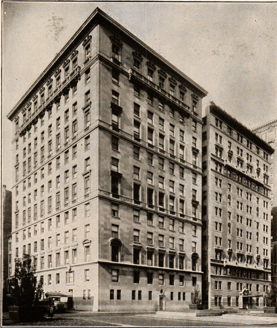
Apartment Building, Park Avenue, New York City. Warren & Wetmore, Architects. Faced with Indiana Limestone.
