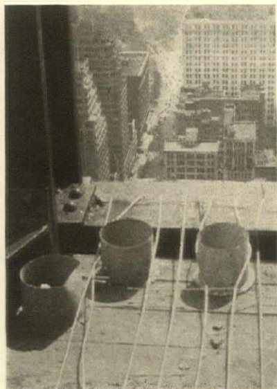
Reinforcing mesh wires spread around sleeves, with adjoining cross wires cut
