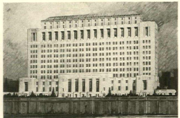
Ohio's proposed State office building in Columbus. Harry Hake, architect; Frank W. Bail, Alfred A. Hahn, consulting architects
