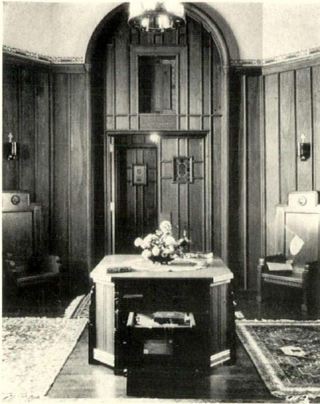
Inside the main reception room, looking toward the main entrance
