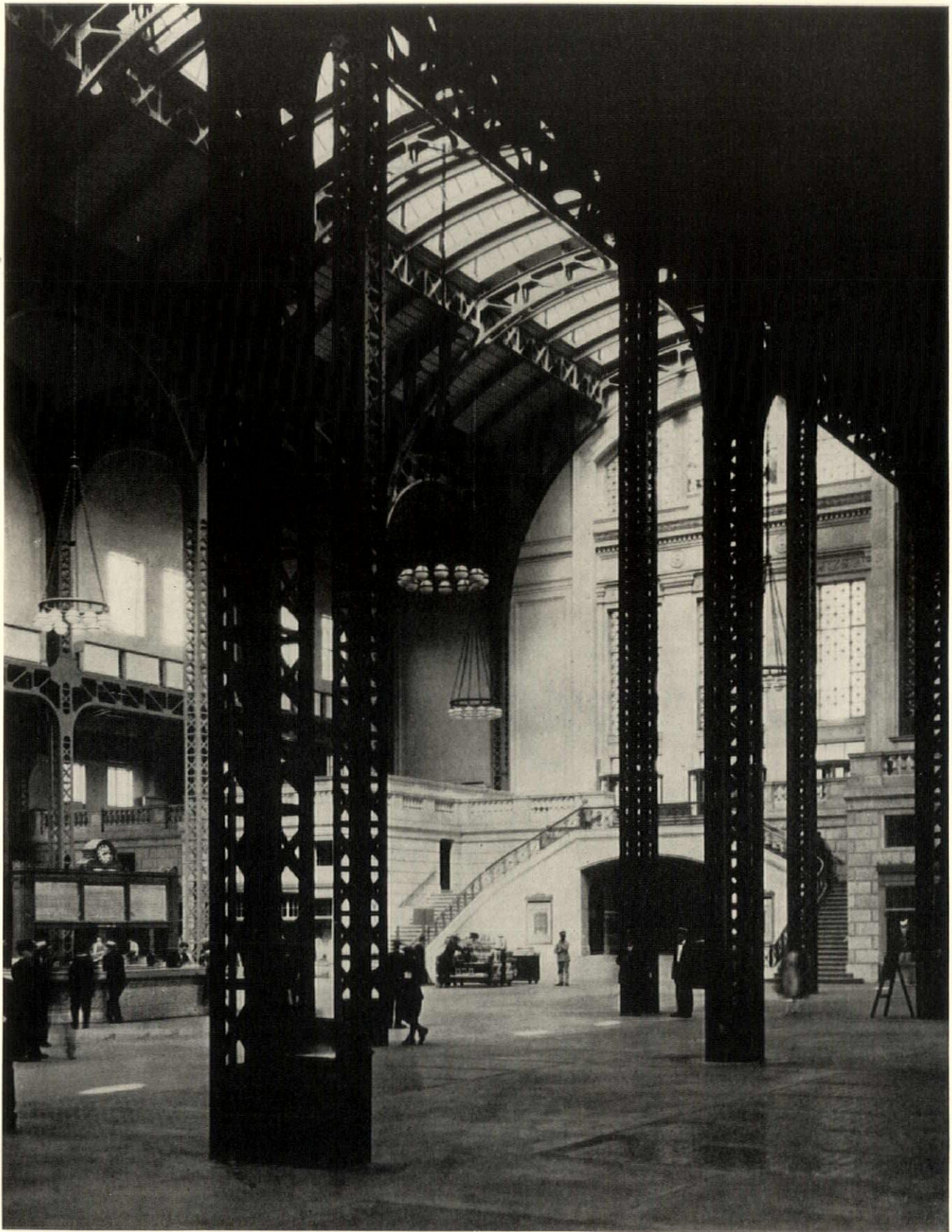
A sensible and beautiful rendering of the functional steel members. Concourse of Union Station, Chicago, Ill. Graham, Anderson, Probst & White, architects
