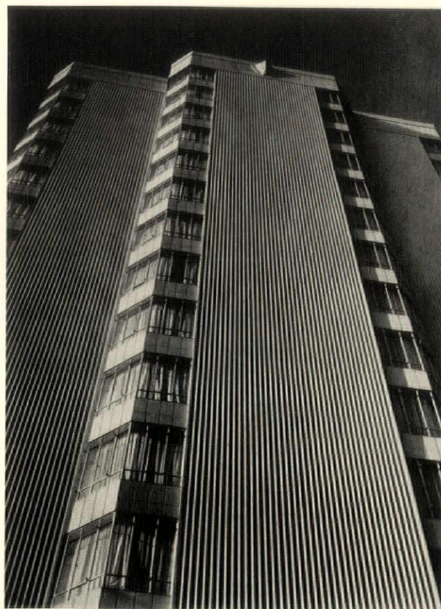
A recent construction in monolithic concrete with no reference to past styles, and entirely dependent upon the limitations and possibilities of its material for any architectural charm it may possess. Edmond Meaney Hotel, Seattle, Wash. Robert C. Reamer, architect
