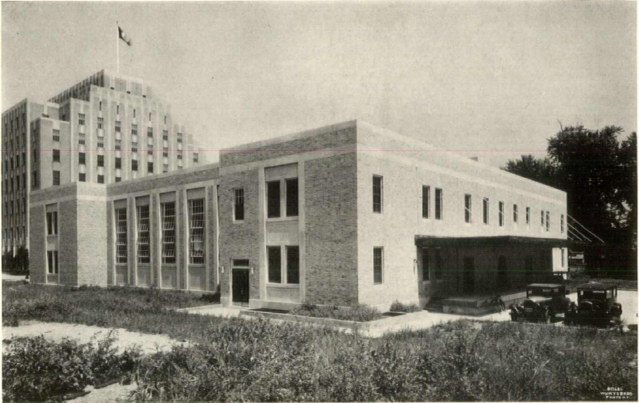
Above, a corner view from the rear, showing at the right the mailing platform. The only part of the building below grade is that under the rear end block, providing for boiler-room space and storage. Below, the workroom, which has a wood wainscot and wood block floor
