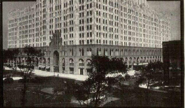
● Fisher Building, Detroit. All heating and cold water lines of Byers Genuine Wrought Iron Pipe.
