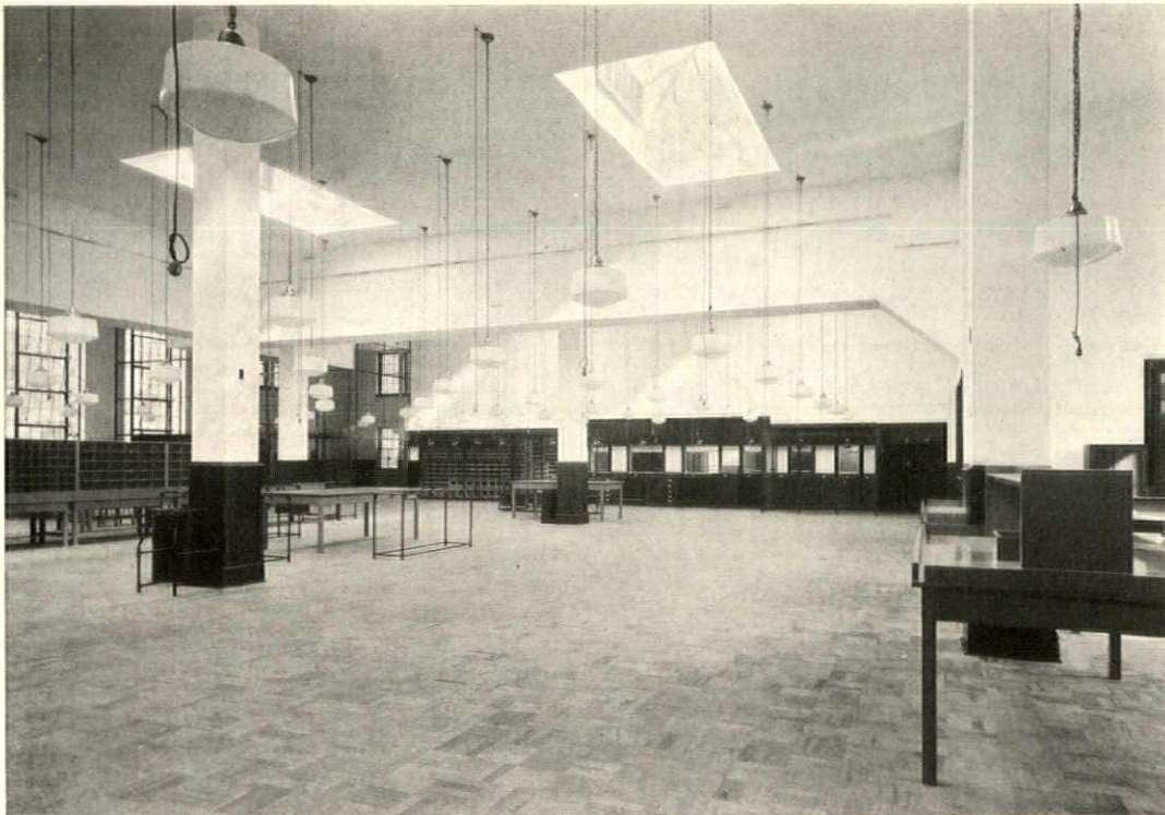
Above, a corner view from the rear, showing at the right the mailing platform. The only part of the building below grade is that under the rear end block, providing for boiler-room space and storage. Below, the workroom, which has a wood wainscot and wood block floor
