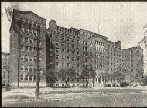
● Byers Genuine Wrought Iron Pipe specified for cold water, hot water, drainage, vents, fire system and all heating lines in Harper Hospital Addition, Detroit.
