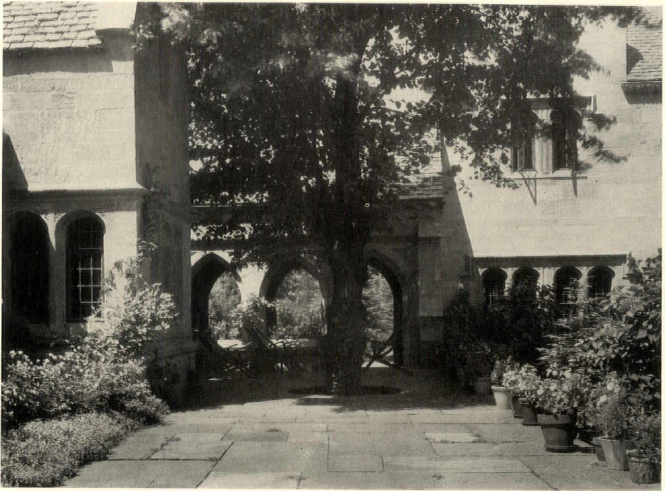
The terrace, which overlooks the garden to the right. In the distance is the cloister joining the two buildings. A graduated heavy slate has been used for the roofs
