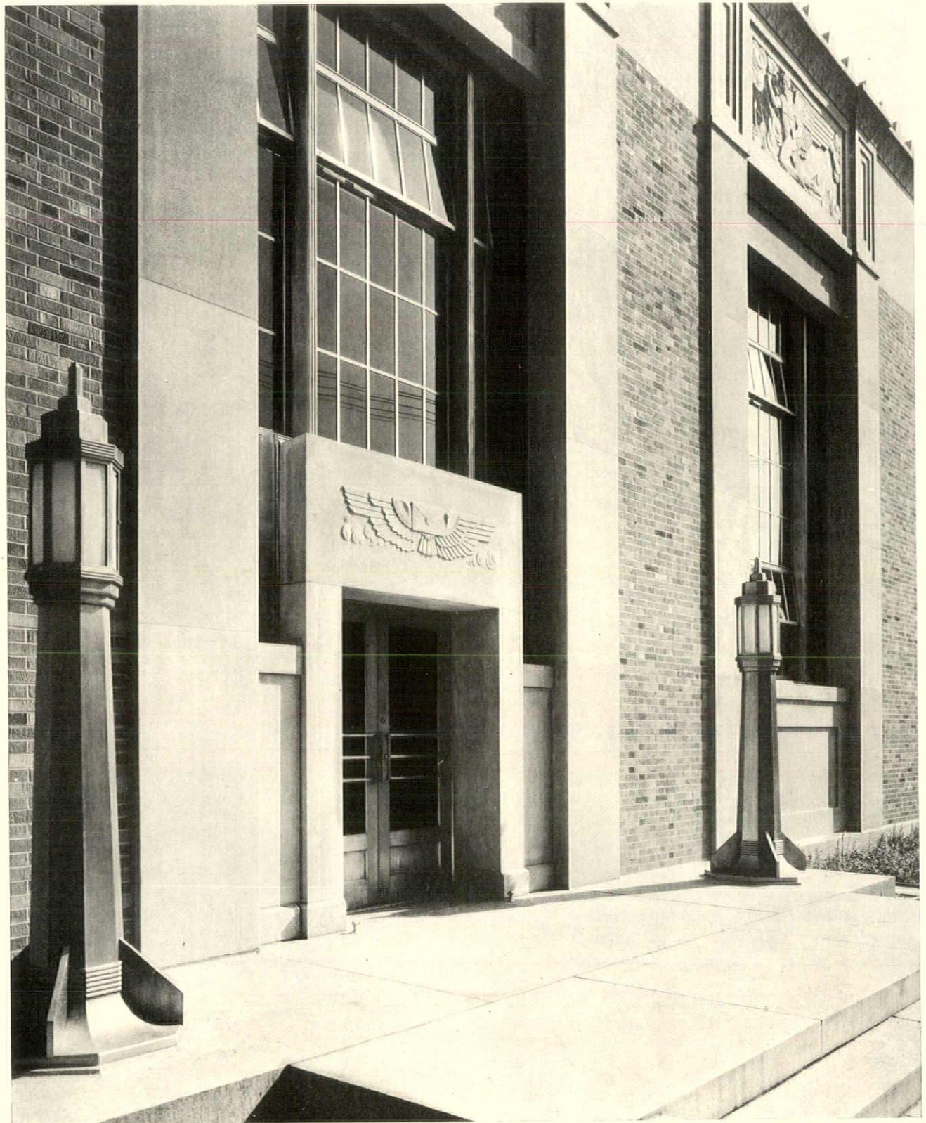
The metal work of the main entrance and the windows across the front of the building are of aluminum, as are also the lighting standards flanking the main entrance. The sculptured panels over the windows, and the abbreviated cornice, are of limestone
