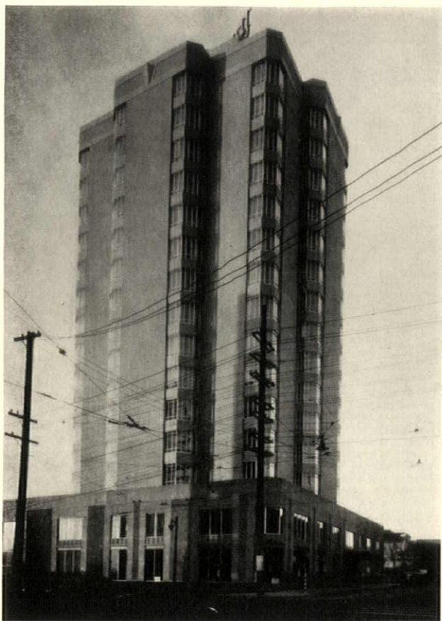
A recent construction in monolithic concrete with no reference to past styles, and entirely dependent upon the limitations and possibilities of its material for any architectural charm it may possess. Edmond Meaney Hotel, Seattle, Wash. Robert C. Reamer, architect
