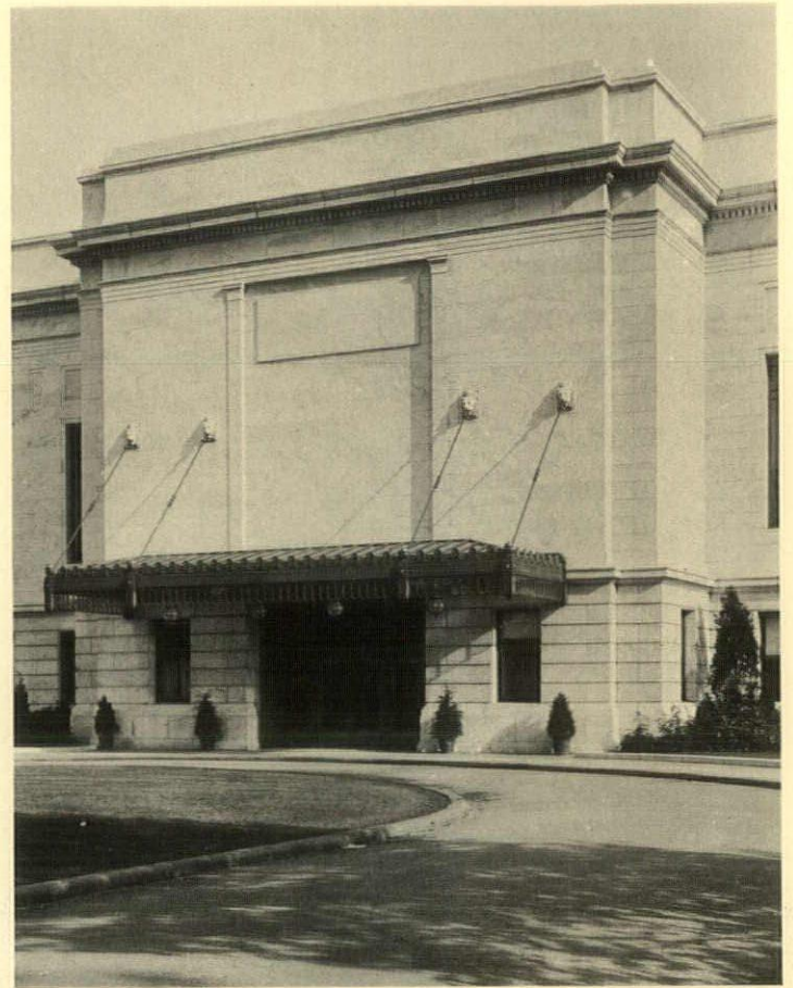
The motor entrance at the ground level
