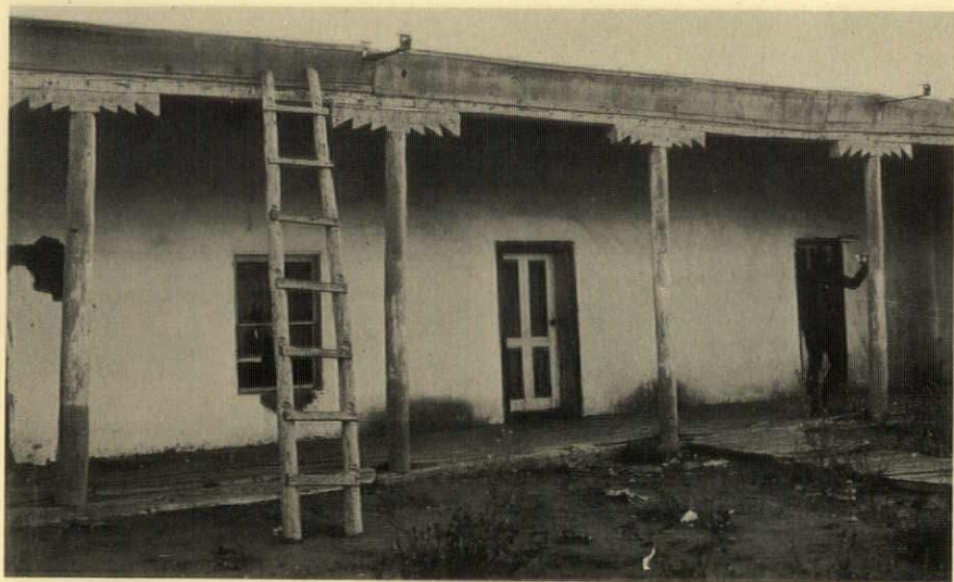
Portal of a house near Alcalde
