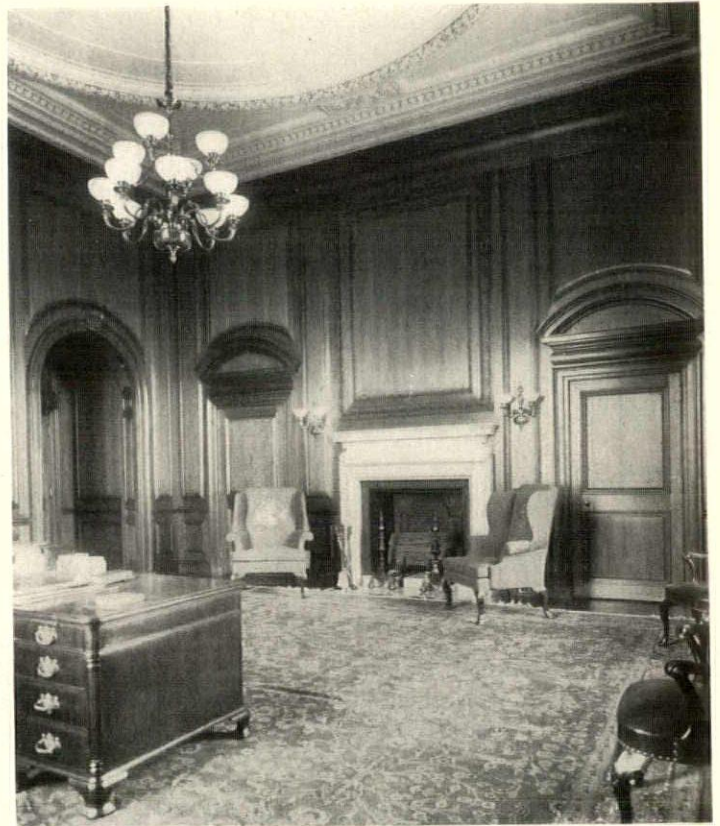
The vice-president's office, the woodwork of which is of walnut in a wax finish, with floor of English oak
