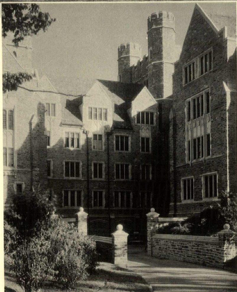
The Medical School, as seen looking down into the service courtyard. The stone used throughout the group is a warm yellow color, quarried from the nearby hills, trimmed with varying buff limestone
