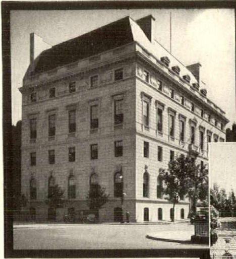
● Genuine Wrought Iron Pipe was specified for waste lines, vents, main soil lines and sewer connections in the Union Club House, New York City.
