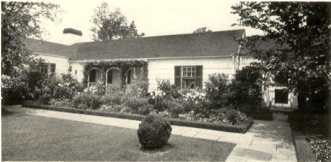
The north wing as seen from the garden court, with the entrance to the kitchen screened by this vine-sheltered porch
