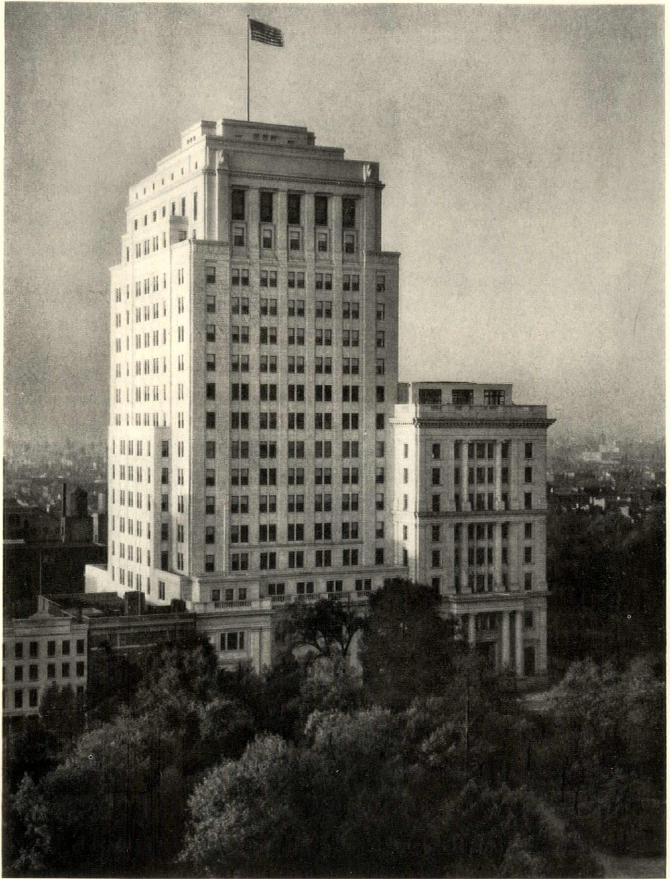
The lower part of the addition follows closely the architecture of the old structure. Beginning, however, with the third story, the walls are set back, avoiding incidentally the robbing of this east side of the old building of its outside light
