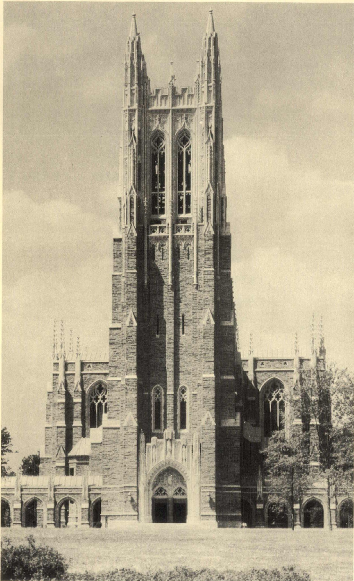
Front view of the Chapel. Its main entrance is on the transverse axis of the campus, always in sight as one approaches through the long driveway
