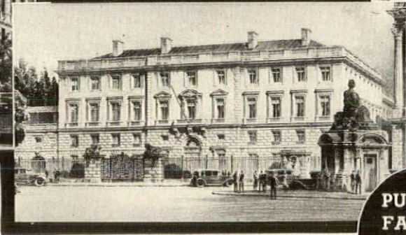
● In the U. S. Embassy, Paris, France, Genuine Wrought Iron Pipe was specified for main plumbing supply, waste lines, vents and drains and heating supply and return lines.
