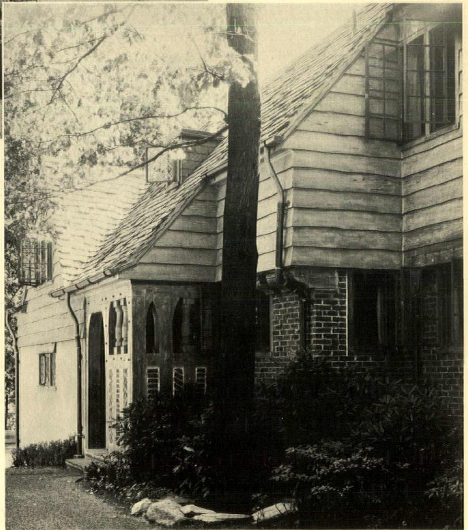
Obviously the exterior was inspired by the houses of the Cotswold district in England. Materials for the exterior were selected with the idea of avoiding maintenance charges so far as possible. The timbers are of solid oak, the siding of rough-sawn pecky cypress
