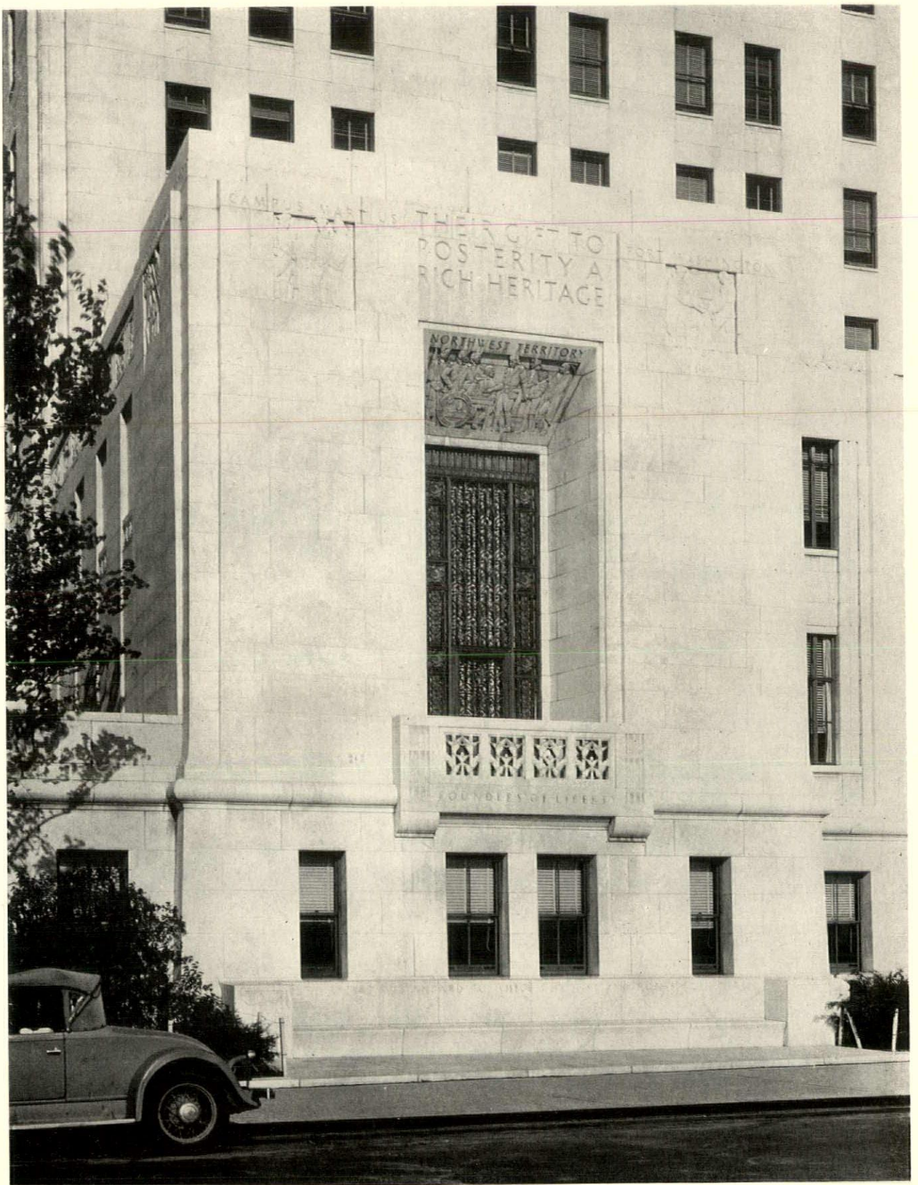
Detail of the north pylon on the river front. Sculpturally this is devoted to the pioneers of the northwest territory, including Boquet's expedition, Fort Washington, Campus Martins, the Greenville treaty, and the establishment of civil government at Marietta
