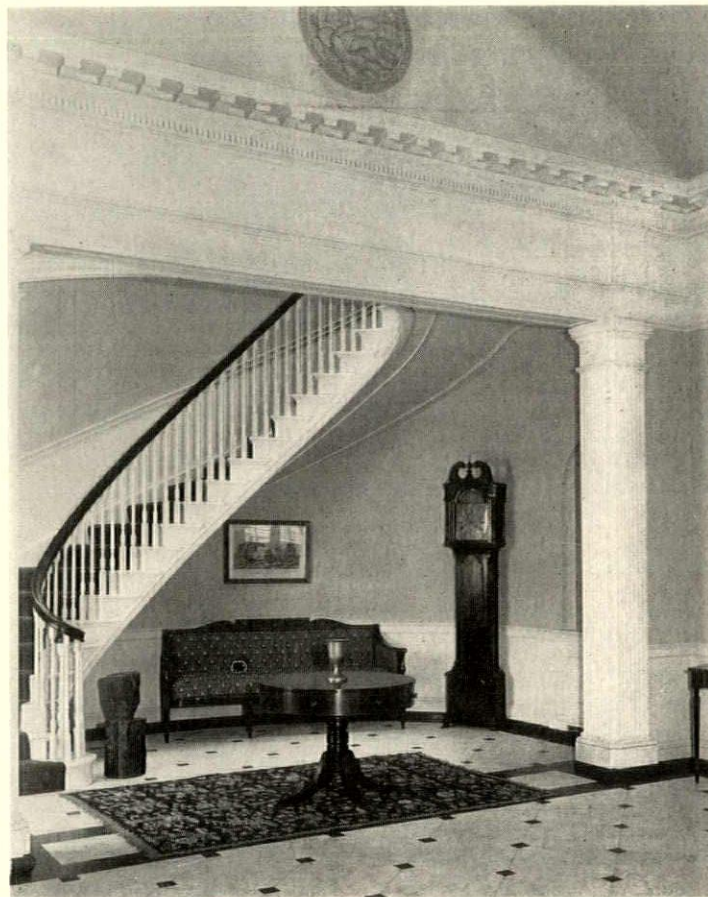
The main staircase at the rear of the entrance lobby. The extreme slenderness of the string is noteworthy
