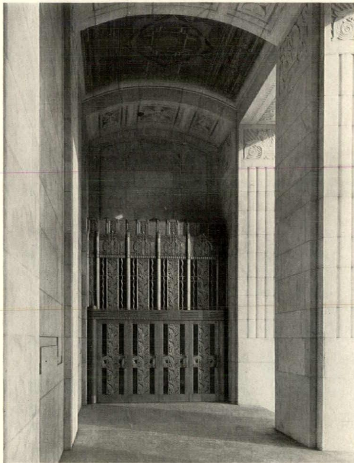
Detail of the Front Street entrance vestibule
