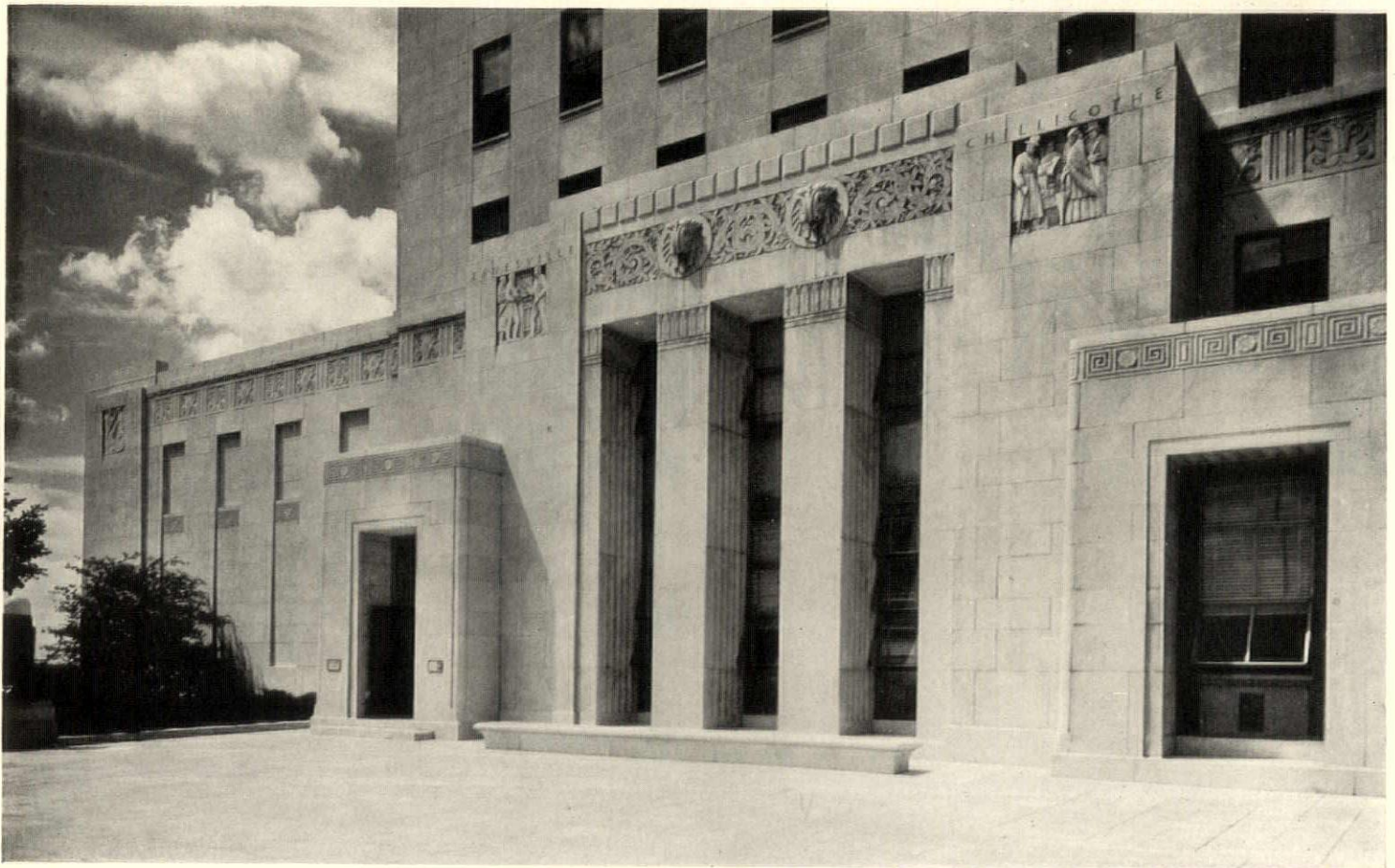
A detail of the south terrace. The two sculptured panels commemorate the former sites of State government
