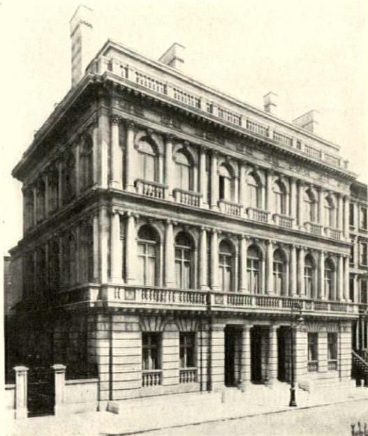
The former New York residence of Joseph Pulitzer—for which McKim, Mead & White were the architects—after having been unoccupied for many years, is to be altered on the interior only, for apartment use
