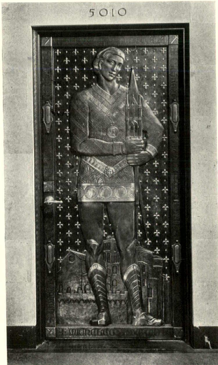
Door to the apartment of Michael Paterno, New York City. Designed and executed by Oscar B. Bach. Bronze repoussé, hand-engraved and enriched with inlays of silver and gold
