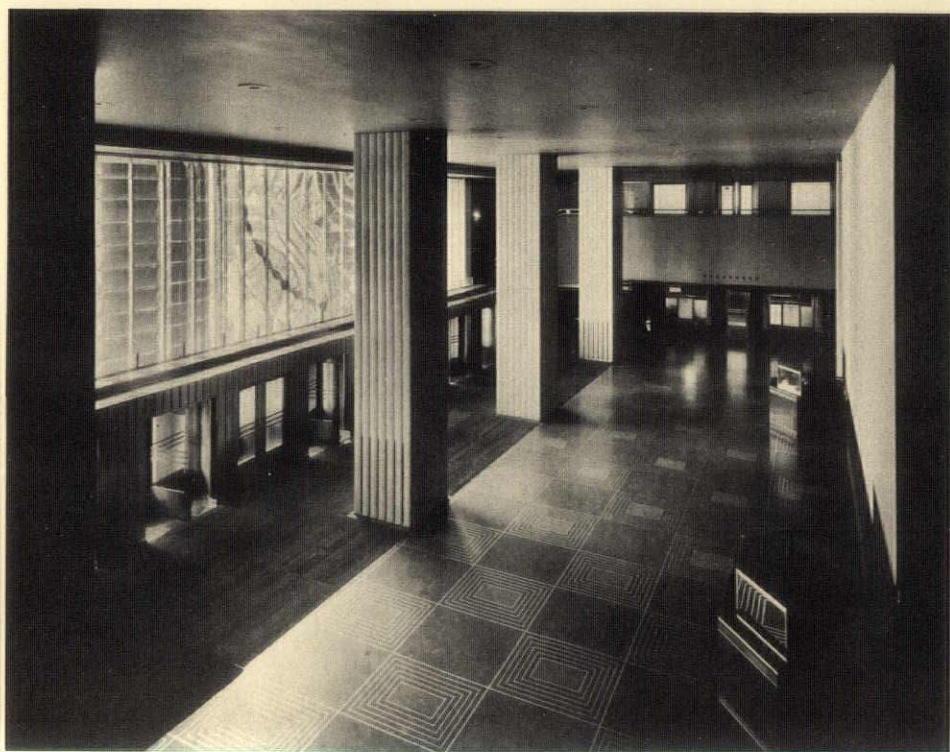
R. C. A. Building, Rockefeller Center, New York City Reinhard & Hofmeister; Corbett, Harrison & MacMurray; Hood & Foulhoux
