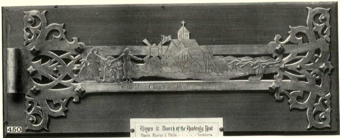
One of a set of hinges for the Church of the Heavenly Rest, New York City. Mayers, Murray & Phillip, architects. Of mild steel, pierced and engraved, with applied bands of the same. Craftsmanship by Bach
