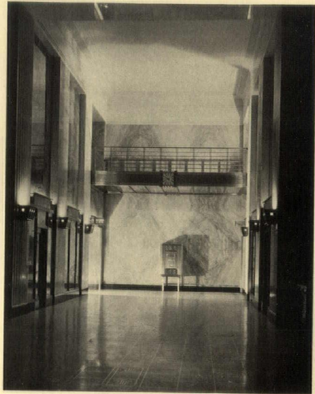
Field Building, Chicago Graham, Anderson, Probst & White
