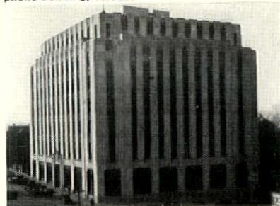
• In the Ohio Bell Telephone Building, Akron, Genuine Wrought Iron specified for hot and cold water, gas, downspouts and vents.
