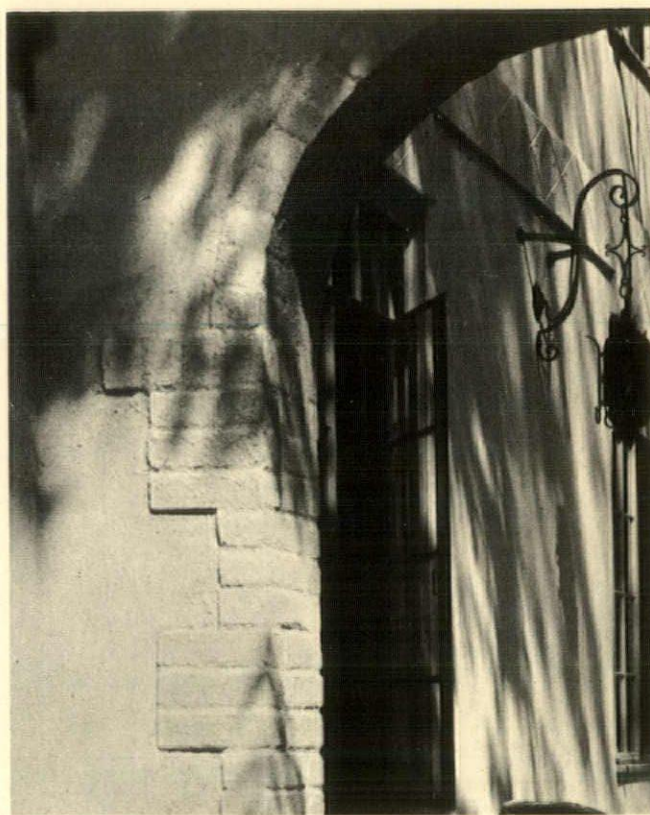
Skim coat of stucco over brick quoins Henry H. Saylor
