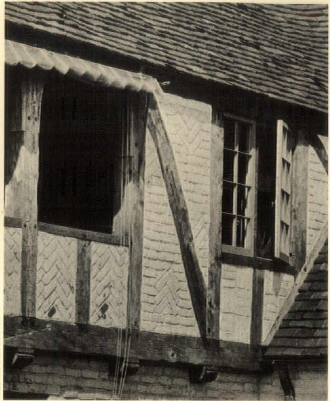
Stable and garage, Greenwich, Conn. Greville Rickard
