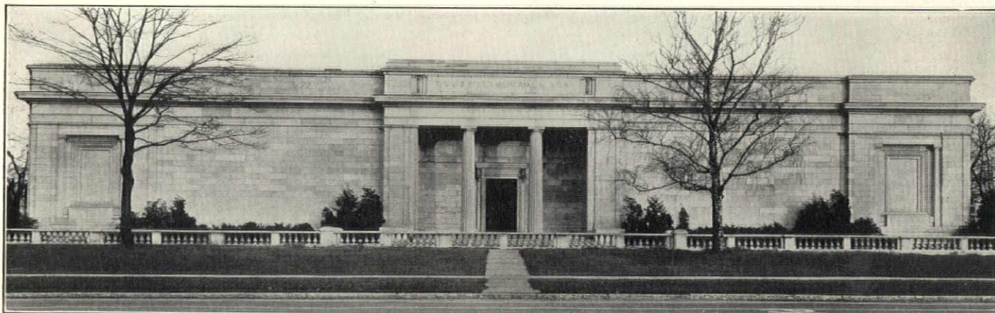
Art Museum of the J. B. Speed Memorial, Louisville, Ky., protected with a Genasco Standard Trinidad Built-up Roof since 1926. Arthur Loomis, Architect; Wm. A. Netherland, Associate.
