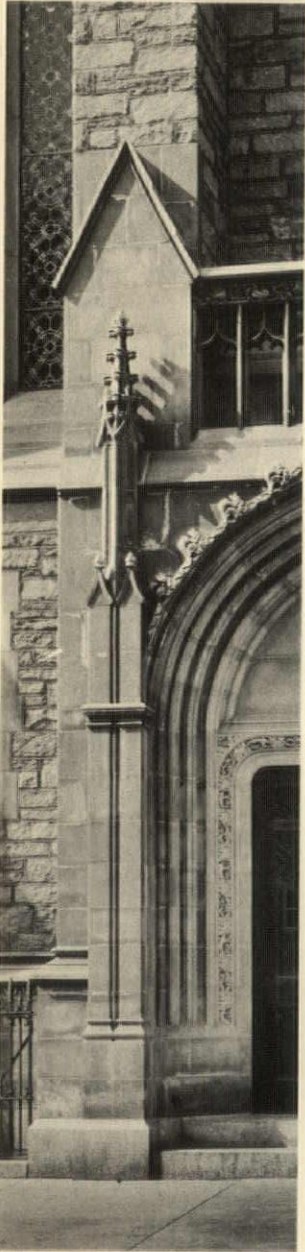
Park Avenue Baptist, Church, New York City Henry C. Pelton; Allen & Collens
