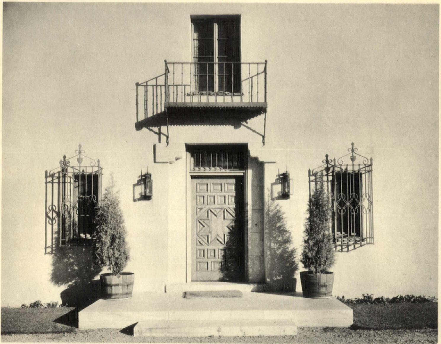
The entrance doorway, true to the chief characteristic of the simpler Spanish prototypes, in that what ornament is used is made to count by concentration against plain wall surfaces of great extent and assymetrical form
