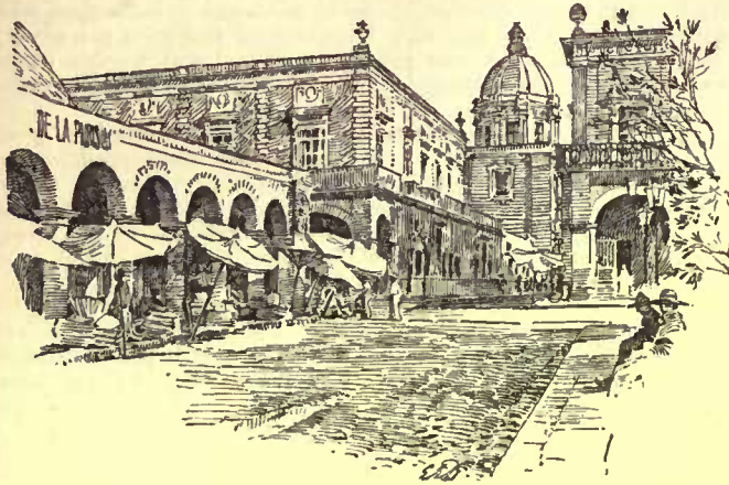
A Corner of the Plaza, Celaya.
