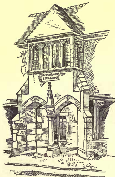
Bay Window in Cloister of Cross, Winchester, Eng.
