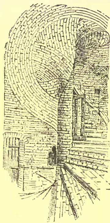
Staircase · House of Tristan the Hermit · Tours · France
