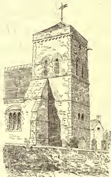
TOWER OF OLD CHURCH. WESTON FAVELL, ENG. AFTER SKETCH BY THOMAS GARRATT. AA ARCH. BOON. LONDON
