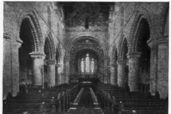
Nave, looking West.
