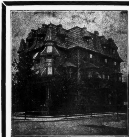
A PHILADELPHIA RESIDENCE ROOFED WITH 14 OZ. COPPER "SPANISH TILES."
