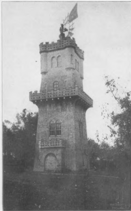
Water-tower, Primrose Park, Mt. Vernon, N. Y. Mr. Frank Marion Wright, Architect.
