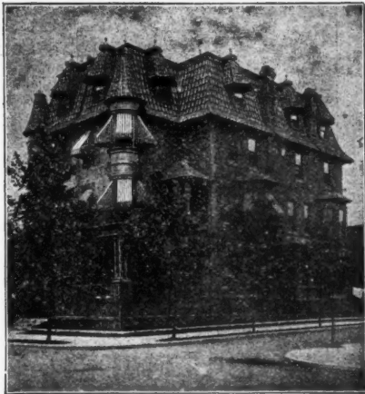
A PHILADELPHIA RESIDENCE ROOFED WITH 14 OZ. COPPER "SPANISH TILES."
