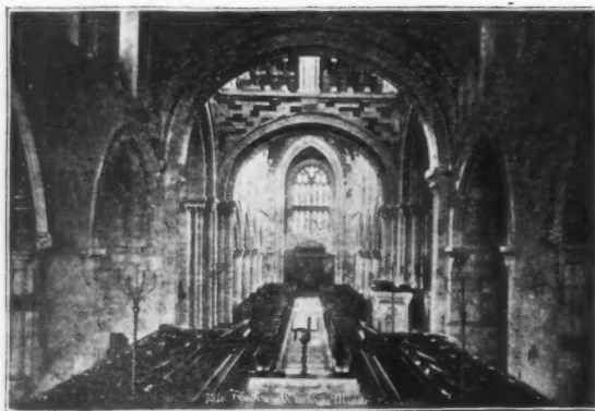
Nave, looking East.
