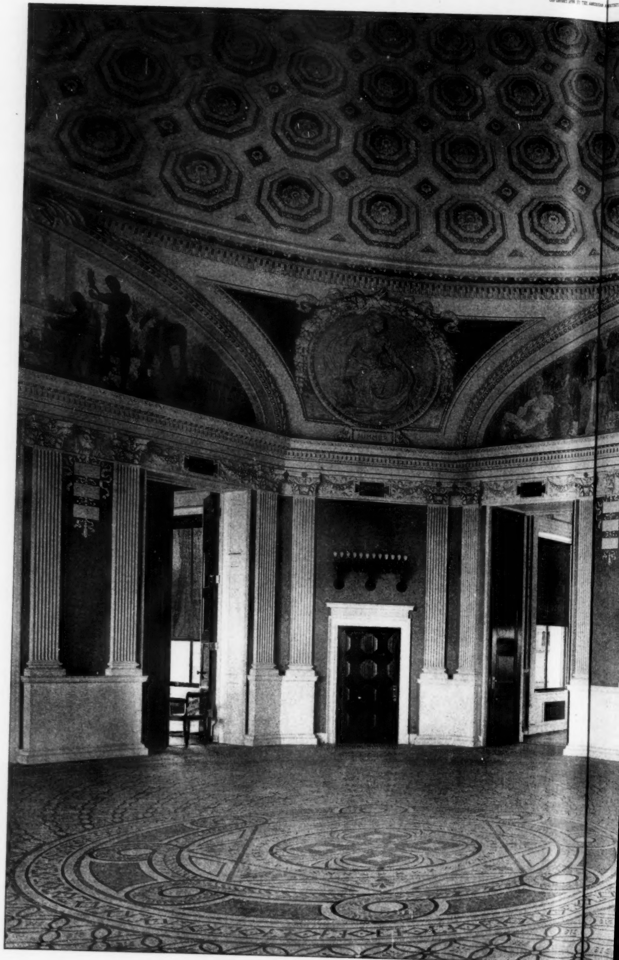
NORTHWEST PAVILION: LIBRARY OF ARCHITECTS: SMITHMEYER & PELZ;
