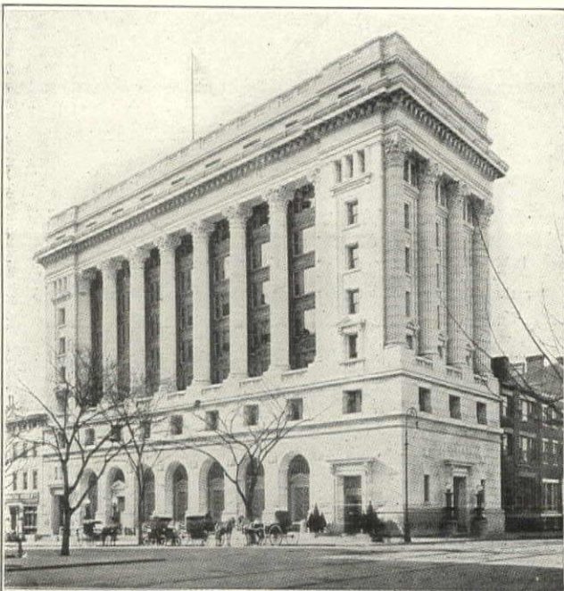
Union Trust Co. Building, Washington, D. C. Wood, Donn & Deming, Architects.
