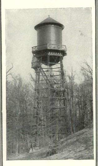
WE make a specialty of the design and construction of steel tanks for fire protection and general service. Our elevated tanks give a positive direct supply of water under pressure which is independent of the operation of any machinery to maintain the pressure until the tank is entirely empty.
