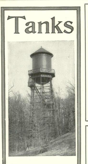
W<sup>E</sup> make a specialty of the design and construction of steel tanks for fire protection and general service. Our elevated tanks give a positive direct supply of water under pressure which is independent of the operation of any machinery to maintain the pressure until the tank is entirely empty.
