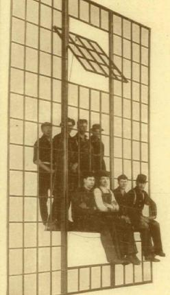
Remarkable Strength of United Steel Sash. Eight Men Balanced on Ventilator.
