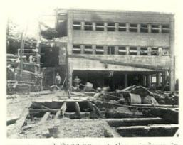
An expenditure of \$15.00 restored the concrete, and \$132.00 put the windows in good condition. A few days after the fire the representatives of the Insurance Companies held a banquet in the concrete building to adjust the loss on the plant. Within a week after the fire, the owners ordered their architects to design three more concrete factories.
