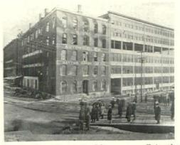
When the fire started in the upholstery department on the fourth floor of the concrete building at the right, it had been completed so recently that automatic fire doors had not been installed nor had the sprinkler system been connected to the water supply. After gutting this floor, the fire spread to a first class mill-construction building adjoining where the roof, fifth and fourth floors fell in a charred mass and wrecked the building. Although the
