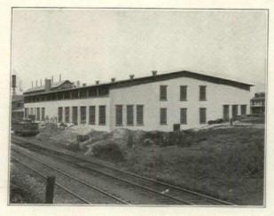
Foundry Building for Bessemer Gas Engine Co. Grove City, Pa. Trussit used for side walls and roofs
