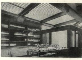
The "Sun Burst" system of Vault Lighting as shown in the illustration, gives a flood of pure white daylight in every corner of the basement. The entire area contains 100 per cent. under-surface of glass and eliminates
