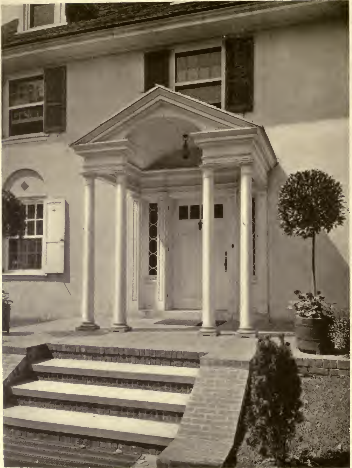
DETAIL OF PORCH
