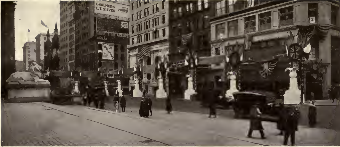
LOOKING NORTHEAST ON FIFTH AVENUE FROM THE TERRACE OF THE PUBLIC LIBRARY.
