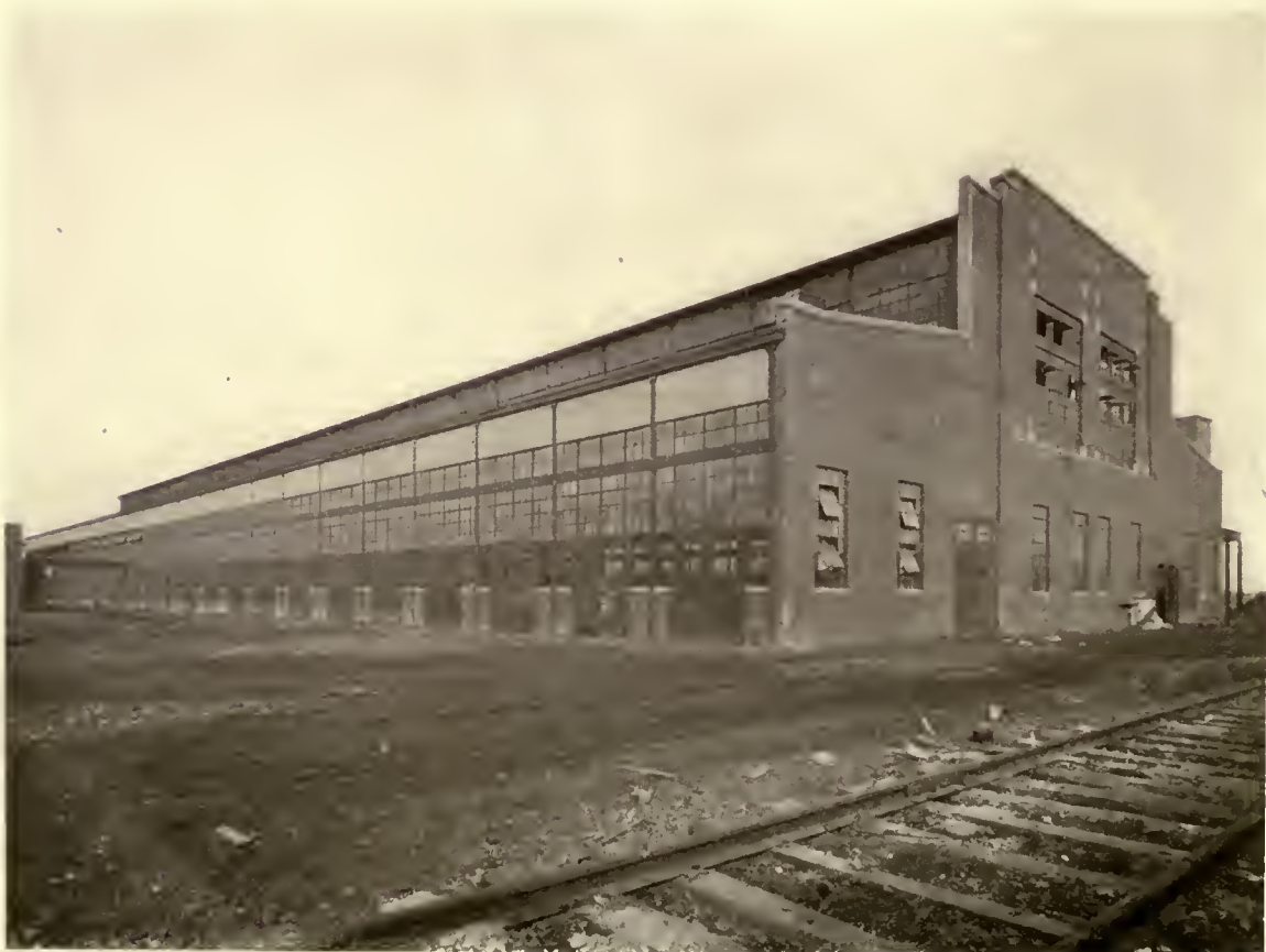
FOUNDRY BUILDING, DODGE BROS., DETROIT, MICH.
