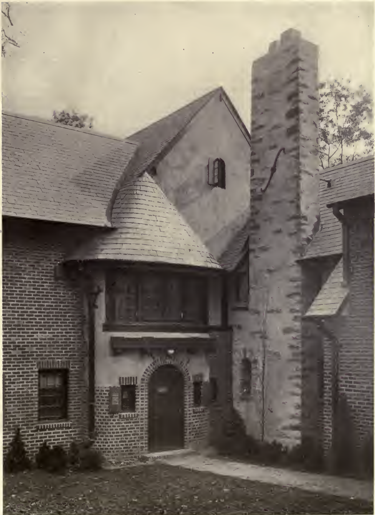
HOUSE OF F. O. ZENKE, ESQ., RIVERALE, N. Y. MR. DWIGHT JAMES BAUM, ARCHITECT
