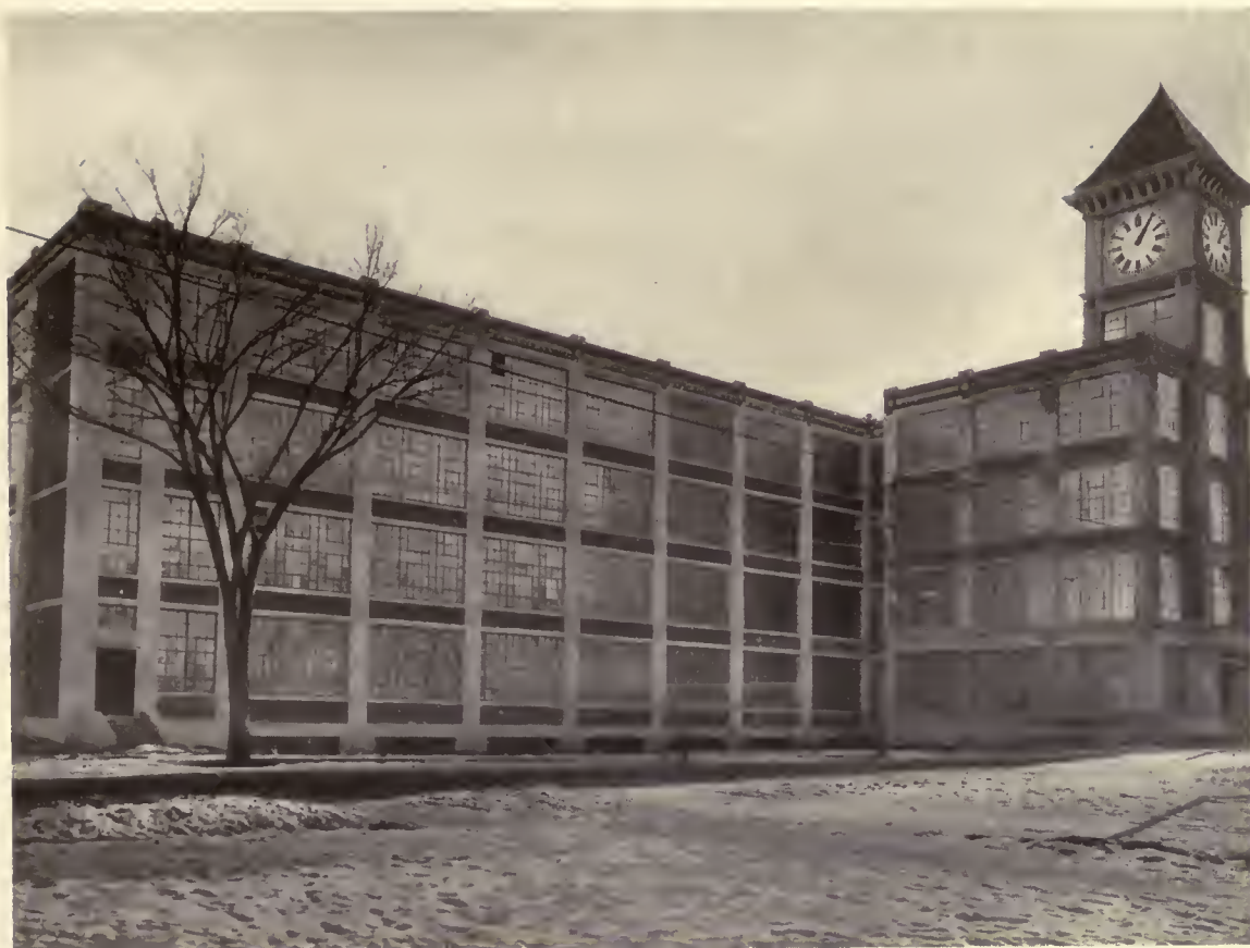
FACTORY, SETH THOMAS CLOCK CO., THOMASTON, CONN. MESSRS. LOCKWOOD, GREENE & CO., ARCHITECTS
