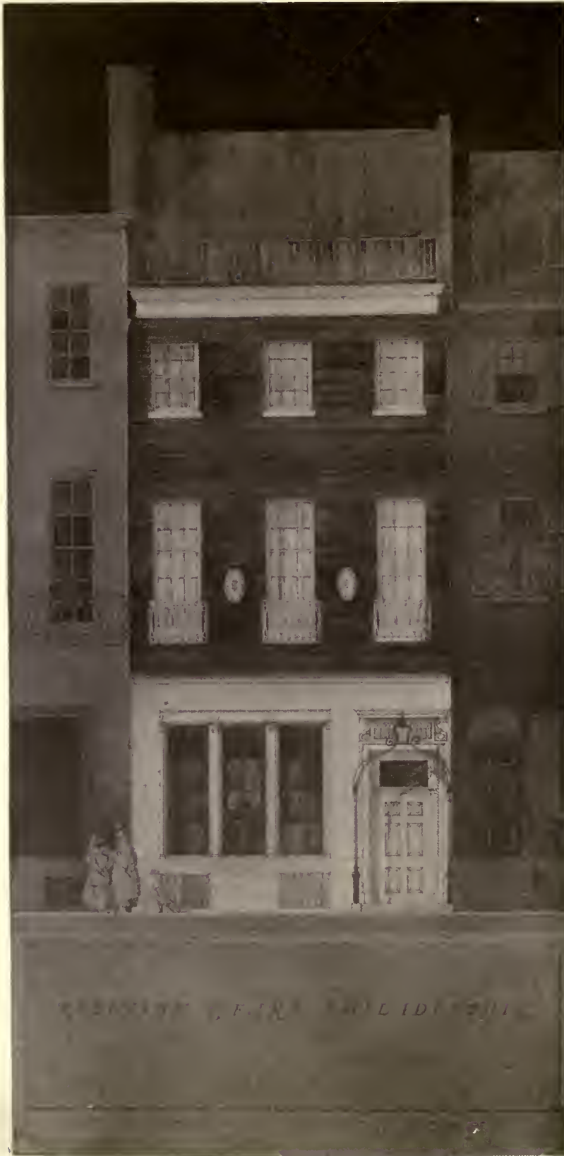
SHOP OF MESSRS. ROBINSON AND FARR, PHILADELPHIA, PA. MESSRS. TILDEN AND REGISTER, ARCHITECTS
