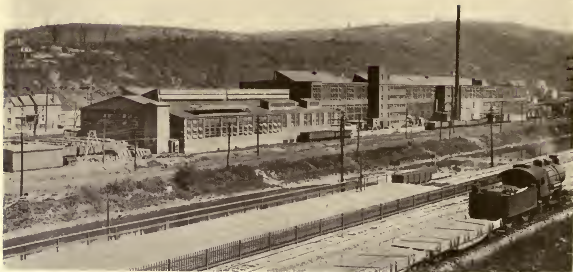
ADDITION TO EAST PITTSBURGH PLANT, WESTINGHOUSE ELECTRIC & MFG. CO.
