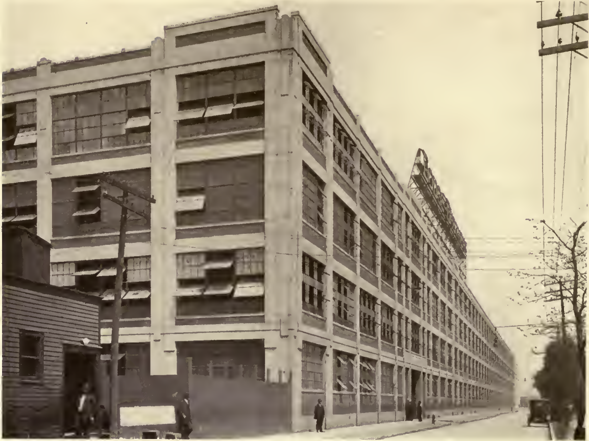
ASSEMBLY BUILDING, DODGE BROS., DETROIT, MICH.
