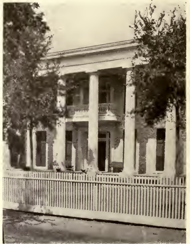
THE NEIL-COCHRAN HOUSE
