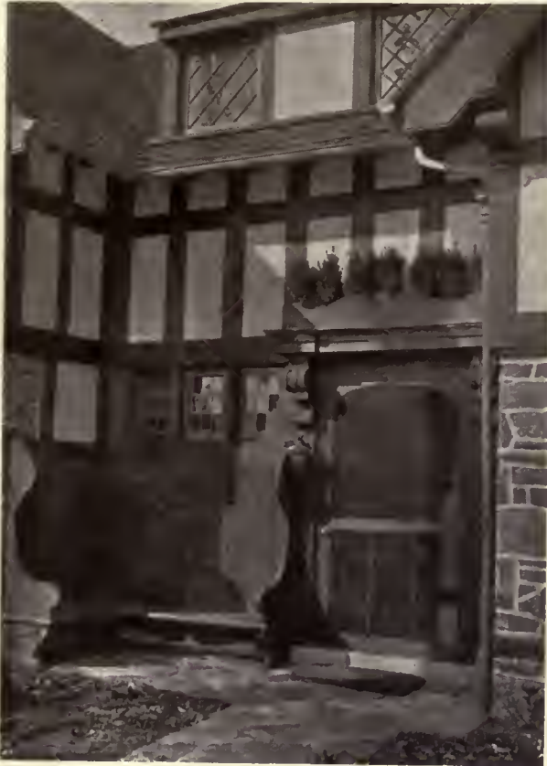
DETAIL OF ENTRANCE—HOUSE OF W. L. MACCOY, ESQ., OVERBROOK, PA. THOMAS H. ATHERTON, JR., ARCHITECT
