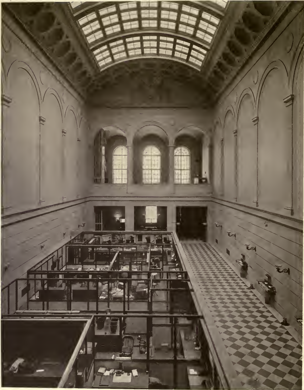
FRANKLIN NATIONAL BANK, PHILADELPHIA, PA. FURNESS, EVANS & CO. AND McKIM, MEAD & WHITE, ASSOCIATE ARCHITECTS
