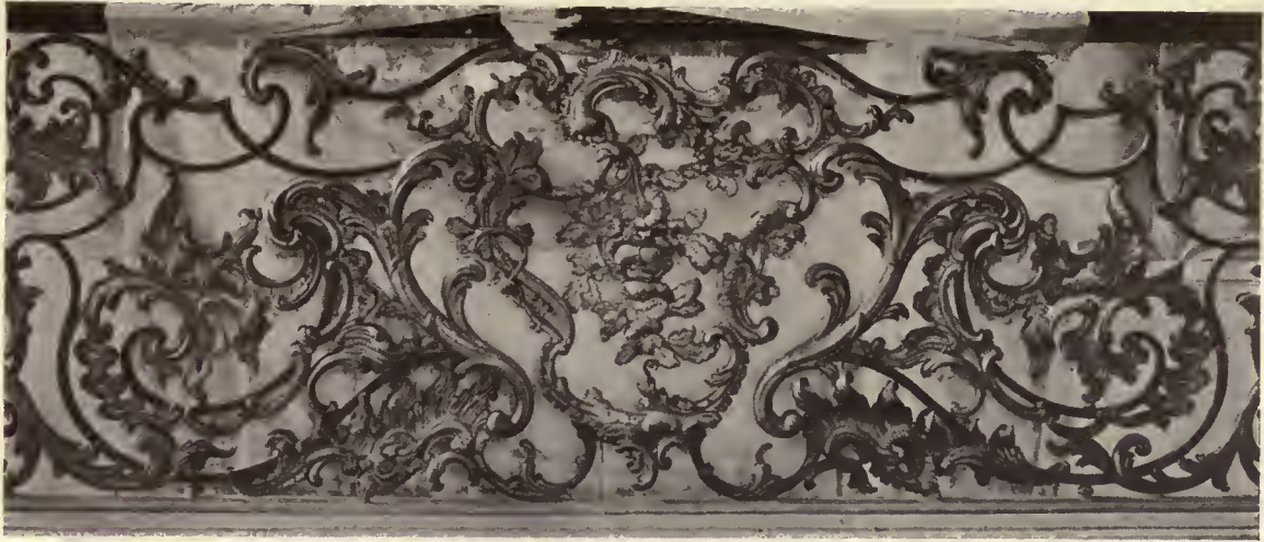
DETAIL OF WROUGHT IRON BALCONY RAIL, HOTEL DE VILLE, NANCY
