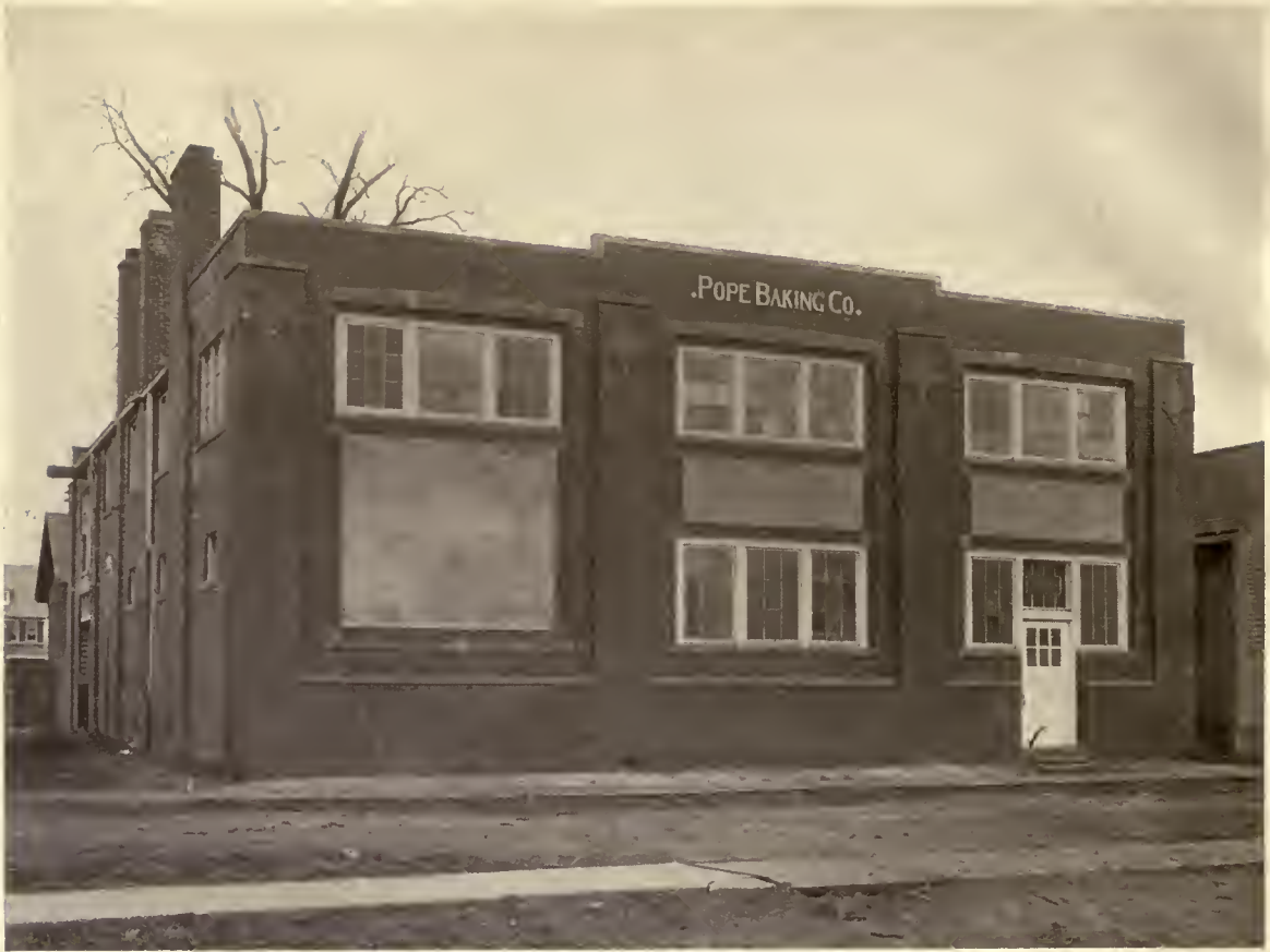
POPE BAKING CO.'S BUILDING, DETROIT, MICH.
