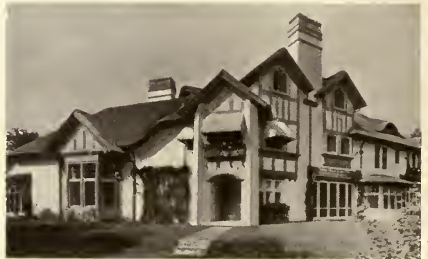
FRONT VIEW—RESIDENCE OF JOHN GLASS, ESQ., HIGHLAND PARK, ILL.
