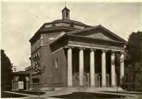
FIRST CONGREGATIONAL CHURCH, TOLEDO, OHIO MILLS, RHINES, BELLMAN & NORDHOFF, ARCHITECTS
