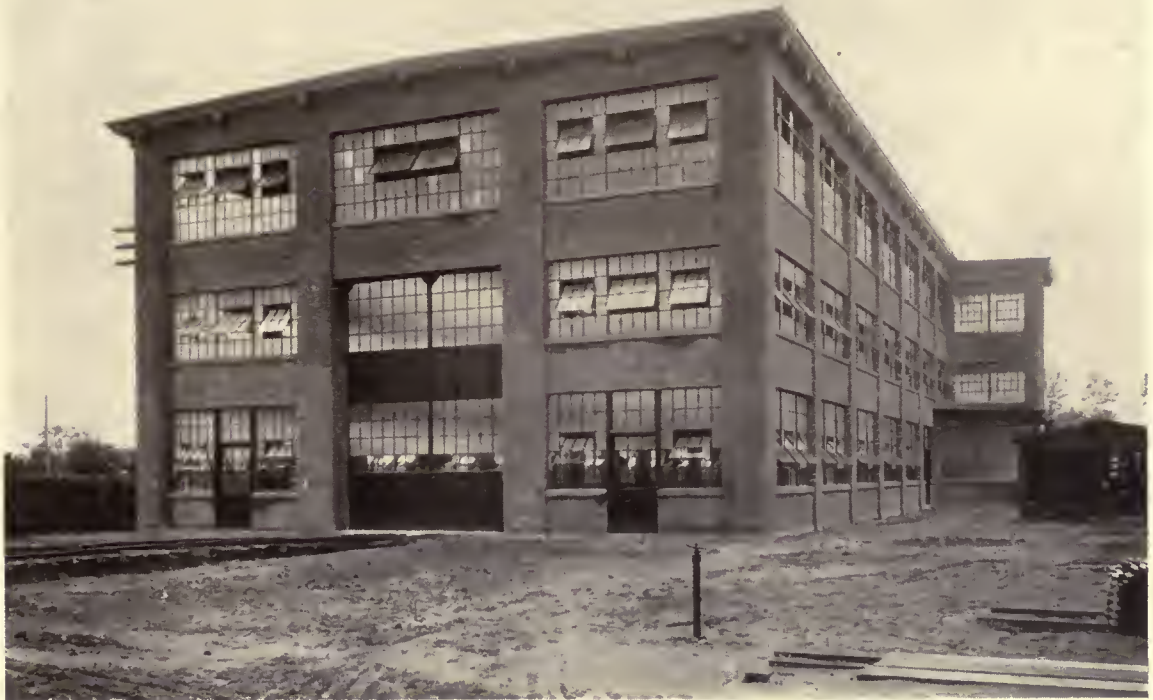
ENGINE ERECTING SHOP, SHEFFIELD CAR CO., THREE RIVERS, MICH. MESSRS. LOCKWOOD, GREENE & CO., ARCHITECTS AND ENGINEERS
