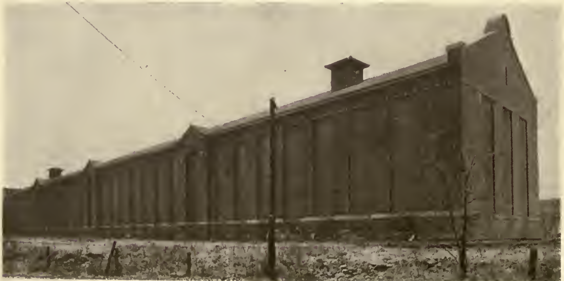
CELL HOUSE FROM OUTSIDE THE WALLS MINNESOTA STATE PRISON GROUP, STILLWATER, MINN. MR. CLARENCE H. JOHNSTON, ARCHITECT
