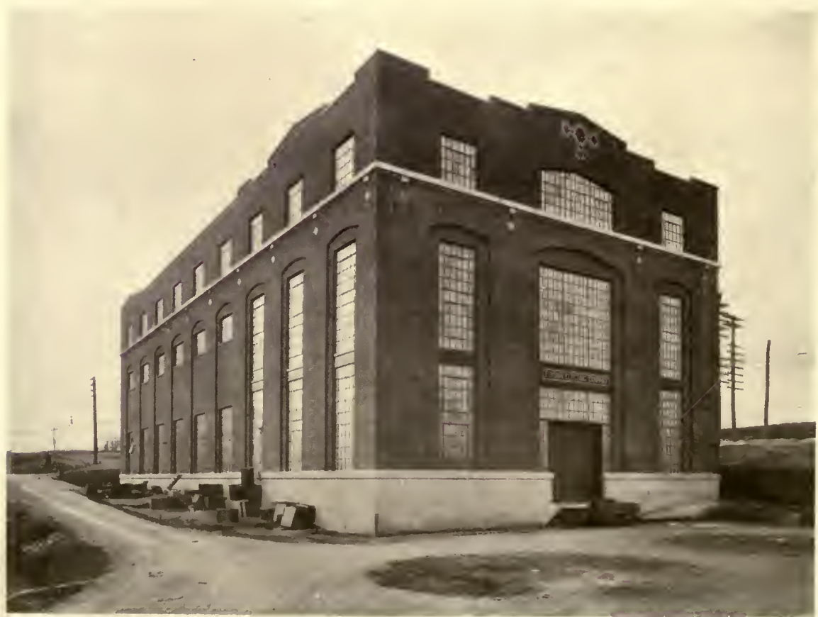
SUB-STATION, EDISON ELECTRIC CO., LANCASTER, PA.
