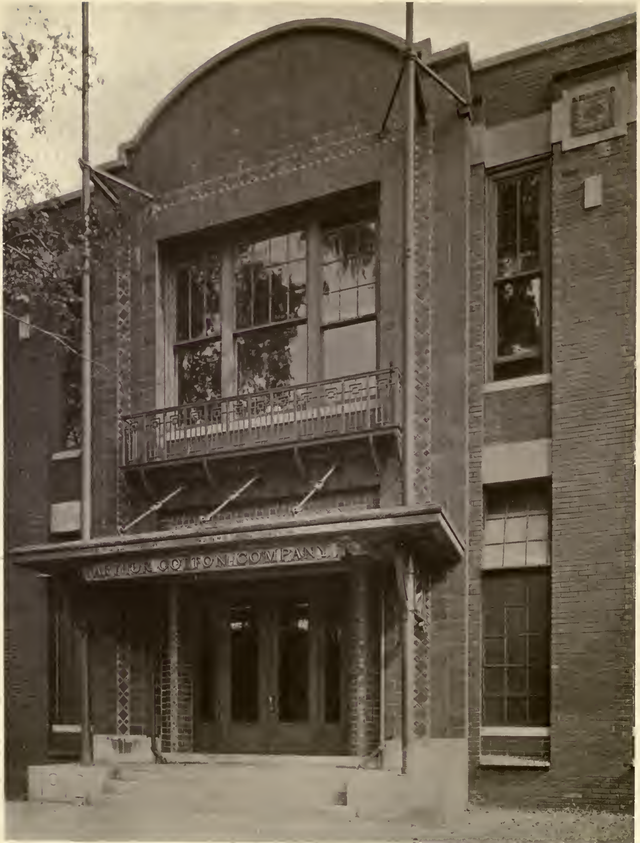
DETAIL OF MAIN ENTRANCE
