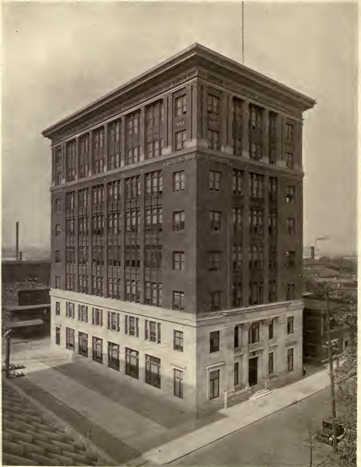
OFFICE BUILDING, VICTOR TALKING MACHINE CO., CAMDEN, N. J. MESSRS. WALTER T. KARCHER AND LIVINGSTON SMITH, ARCHITECTS
