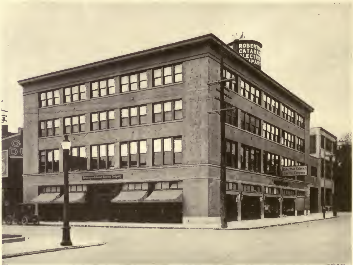
ROBERTSON-CATARACT ELECTRIC CO., BUFFALO, N. Y. MESSRS. WOOD & BRADNEY, ARCHITECTS
