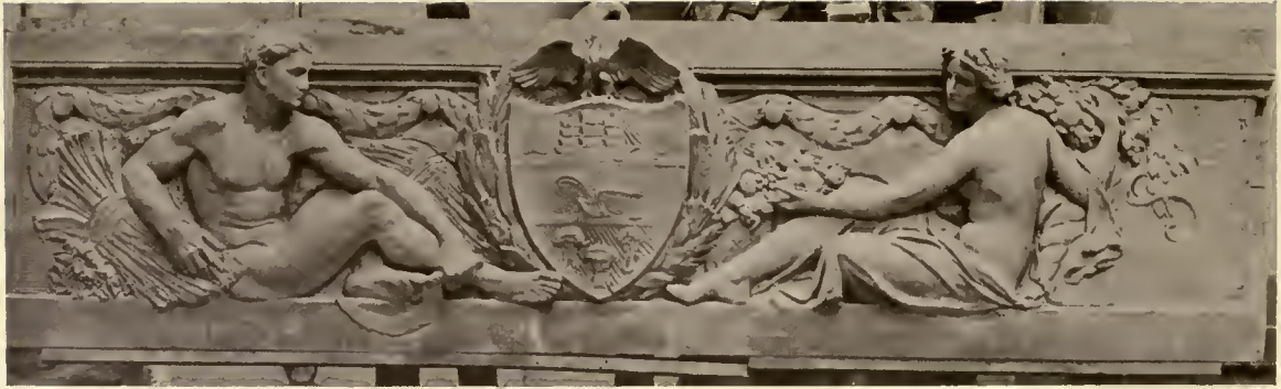
DECORATIVE PANEL, CITY AND COUNTY BUILDING, PITTSBURGH, PA.
