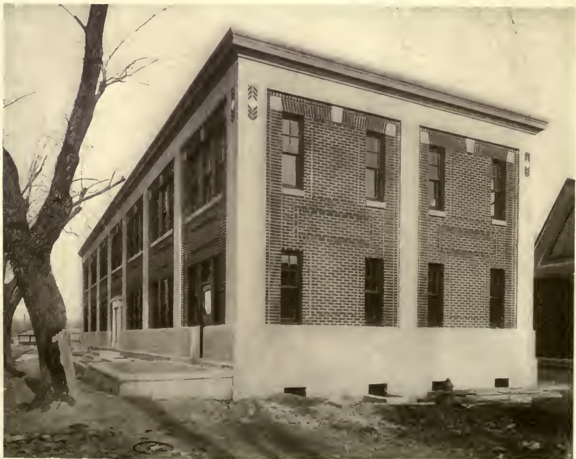
OFFICE BUILDING CINCINNATI-BICKFORD TOOL CO., CINCINNATI, O. MESSRS. DAY & ZIMMERMANN, ARCHITECTS AND ENGINEERS
