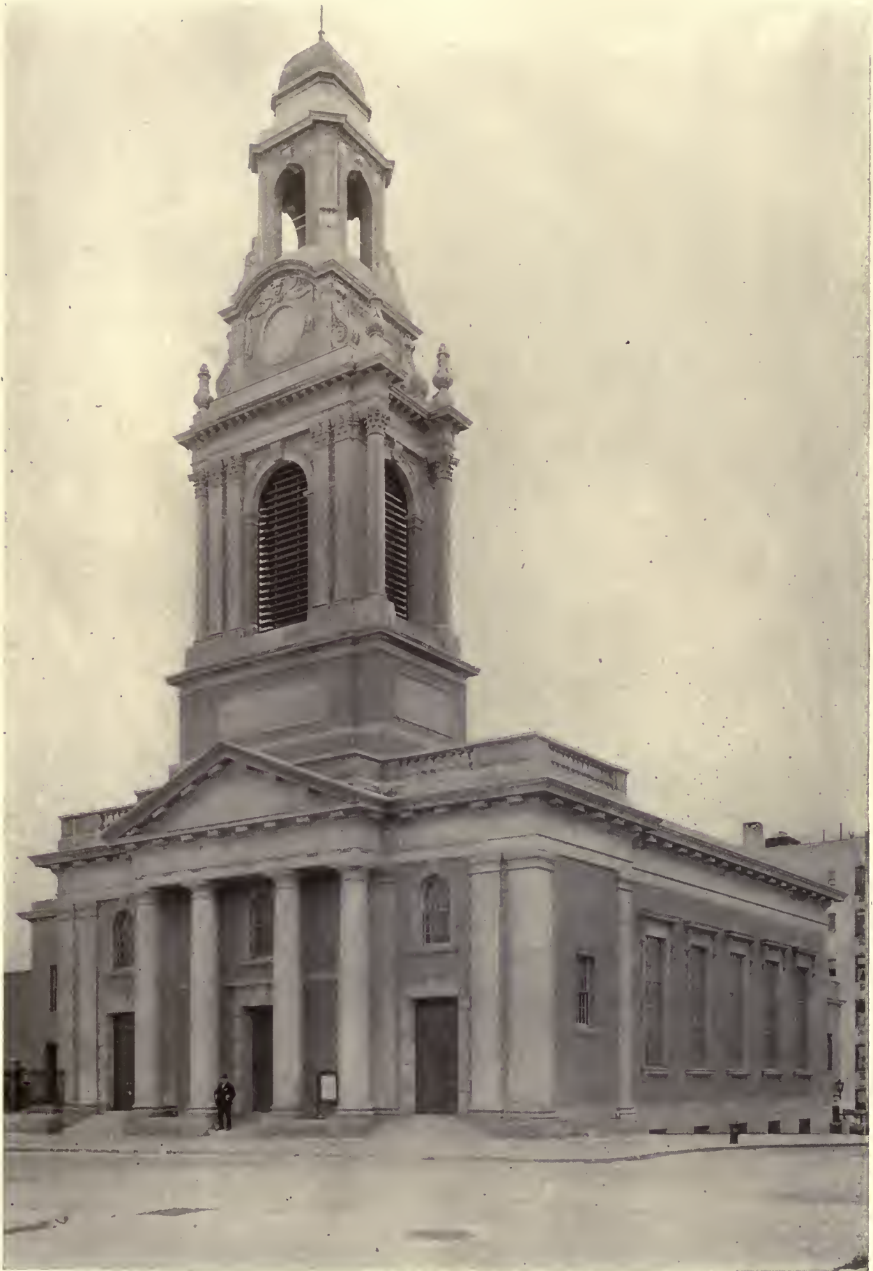
THE FORT WASHINGTON PRESBYTERIAN CHURCH, NEW YORK CITY MESSRS. CARRERE & HASTINGS, ARCHITECTS
