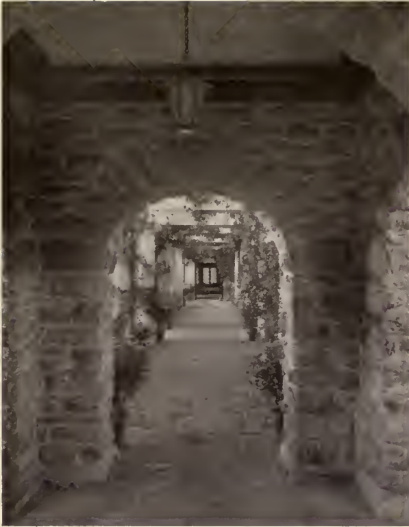
VIEW THROUGH CENTRAL SHELTER LOOKING TOWARD TEA HOUSE
