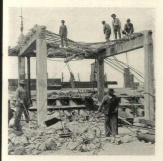
CUTTING SLAB BARS WITH ACETYLENE TORCH
