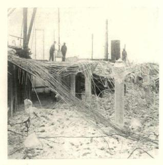
WRECKING FLOOR SLABS WITH BALL
