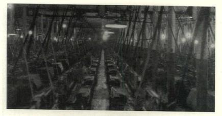
A WEAVE SHOP Poor light due to insufficient number of lamps, their style and location. Very bad glare.
