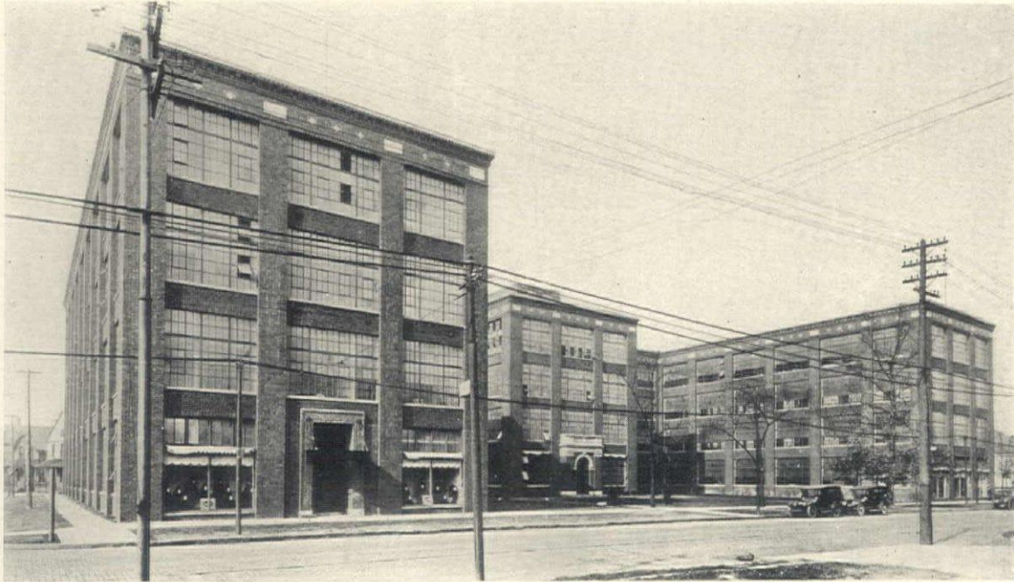
RICHMAN BROTHERS COMPANY FACTORY, CLEVELAND CHRISTIAN, SCHWARZENBERG AND GAEDE COMPANY, ENGINEERS. DANA CLARK, ARCHITECT
