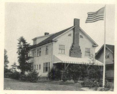
Typical use of wood shingles as siding for a house. They are laid with a wide expanse to the weather.
