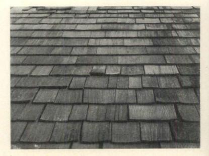
One bundle of shingles on this roof was creosoted. Their location can be seen by the absence of checking and warping. These shingles were laid in 1904 and photographed in 1918. The pitch of the roof is too flat for best results.
