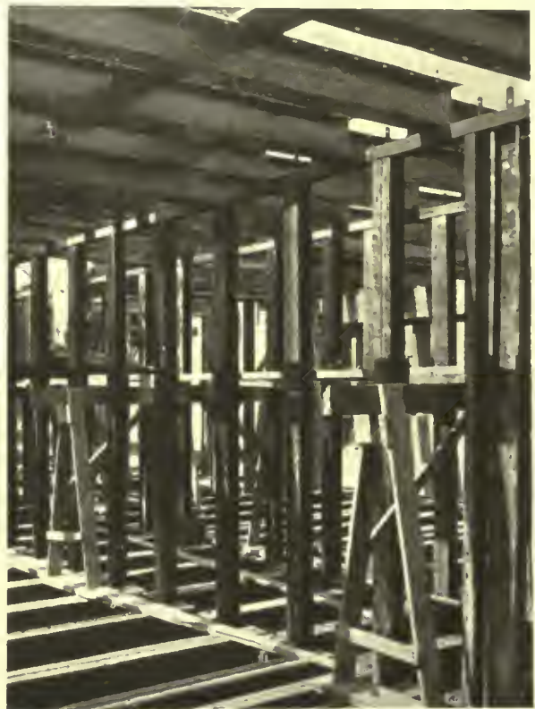
Apartment house construction, showing metal floor joists, studs, cap and sill plates.
