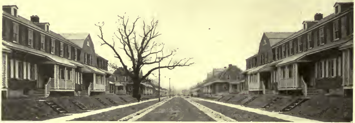
South Philadelphia houses, Essington, Pa. Dubring, Okie & Ziegler, Architects. 200 houses and 1 store building. Work started July 10, 1918; photograph taken Dec. 16, 1918.
