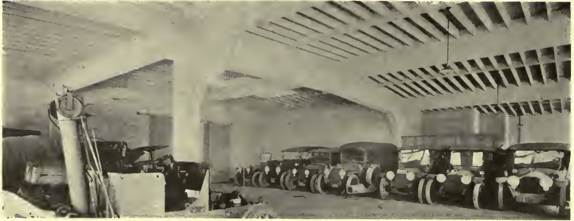
The second floor of the building on the N. W. corner of Second East Street and Social Hall Avenue. This floor is designed for the storage of motor trucks. The construction is of the rigid frame type discussed in the text.
