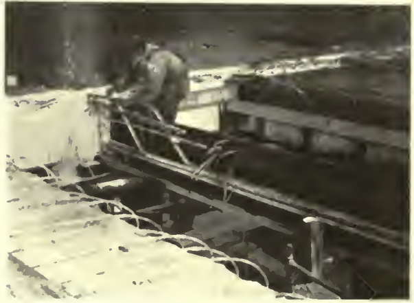
Boxing beam forms around reinforcing rods left in place.
