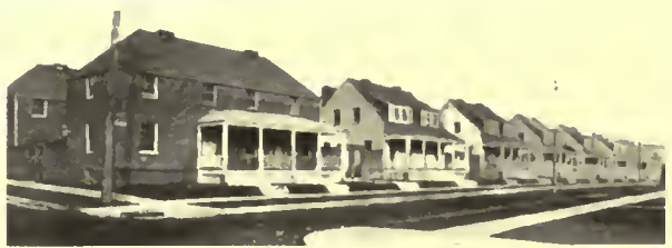
Sun Village, Chester, Pa. Branch of Design, Department of Housing, Architects. 430 houses, 18 apartment buildings with stores under 8. Work started July 12, 1918; photograph taken Dec. 17, 1918. Houses occupied.
