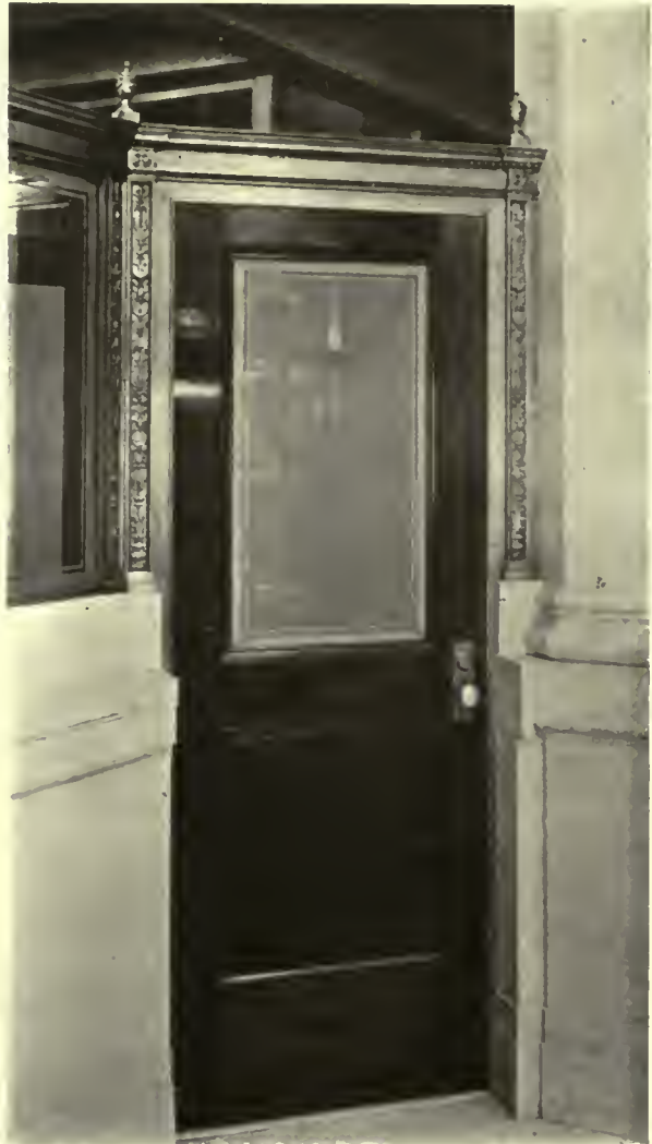
DETAIL OF BRONZE BANK RAILING
