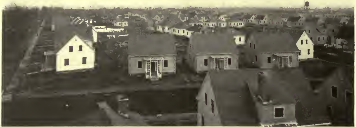
Wyandotte, Mich. Branch of Design, Housing Department, Architects. 78 houses, started Sept. 1, 1918; photograph taken Dec. 16, 1918. Houses occupied.
