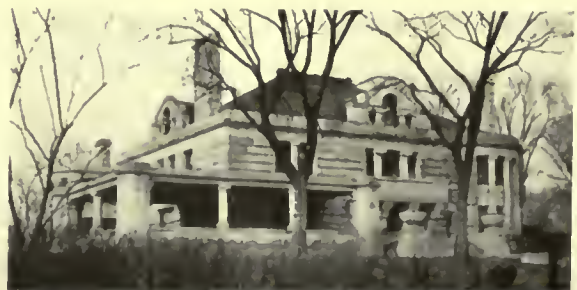
THE CHICAGO SCHOOL. A GREAT HOUSE FOR A CAPTAIN OF INDUSTRY. BUILT IN 1900 GEORGE W. MAHER, ARCHITECT
