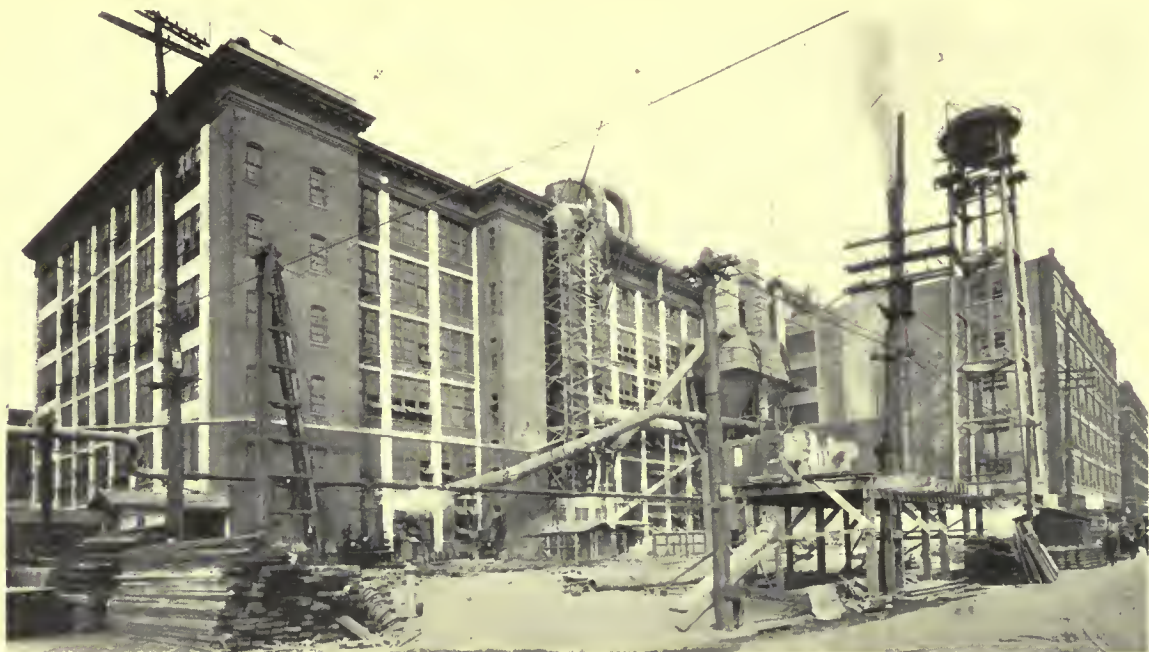
Site of Building 17D, with Buildings 17, 17A at left and center with 17C back of water tower. Building No. 1 at extreme right. Old water tower being wrecked. Note elevated steam main entering at the left and later placed in tunnel.
