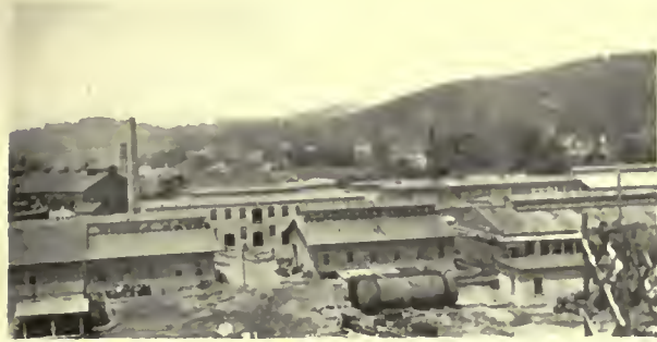
View northwest of Building 1, showing adjoining plant. A typical plant with low buildings, partially combustible and spread out for protection. No special provision for paved roads and economical intra-plant traffic.
