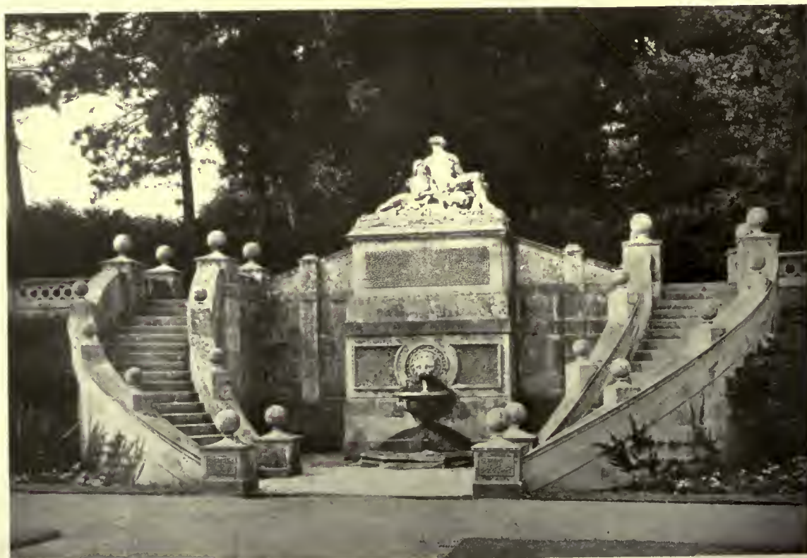
STAIRWAY IN THE GARDEN AT BOXWOOD, WILTSHIRE, ENGLAND
