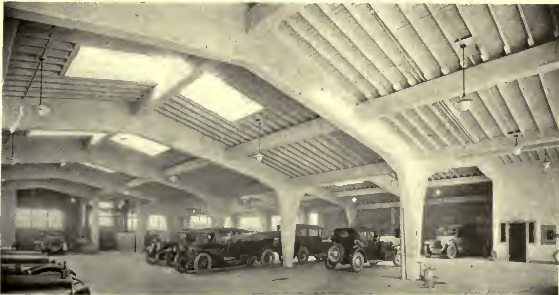
An interior view of the Social Hall Avenue Garage, showing the rigid frame type of reinforced concrete construction.
