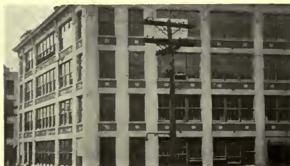
General view of building.
