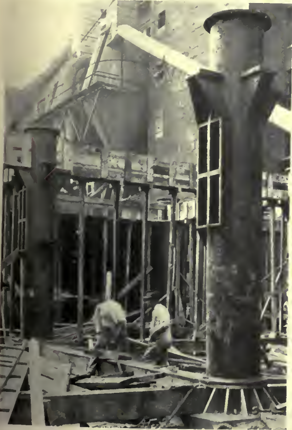
Basement column in position, showing brackets for supporting the floor slab and openings for hot air registers
