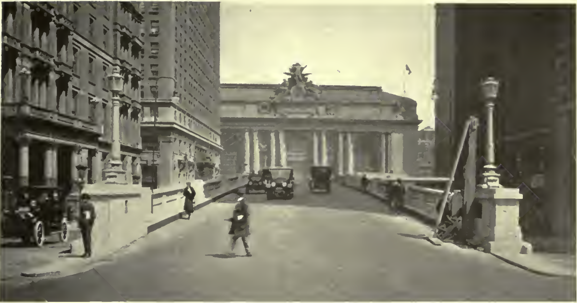
LOOKING NORTH ON PARK AVENUE FROM FORTIETH STREET
