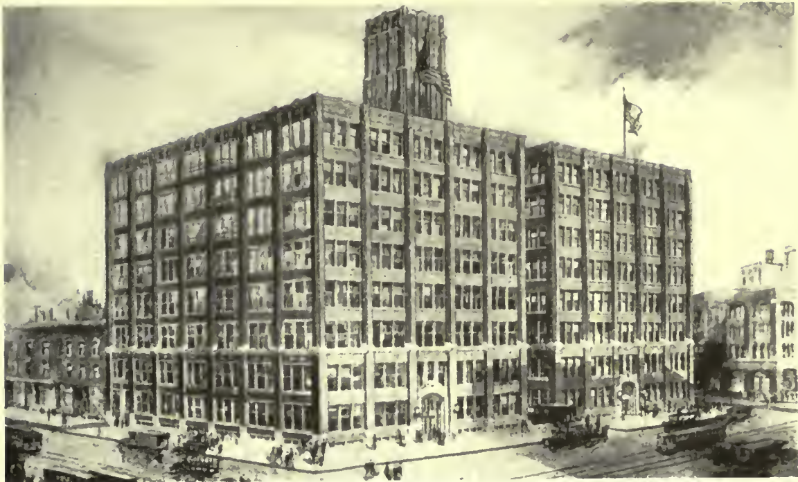
FACTORY, UNION SPECIAL MACHINE CO., CHICAGO GEO. C. SIMMONS & CO., ARCHITECTS
